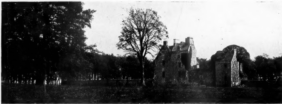
Fig 1.—View from the West.
