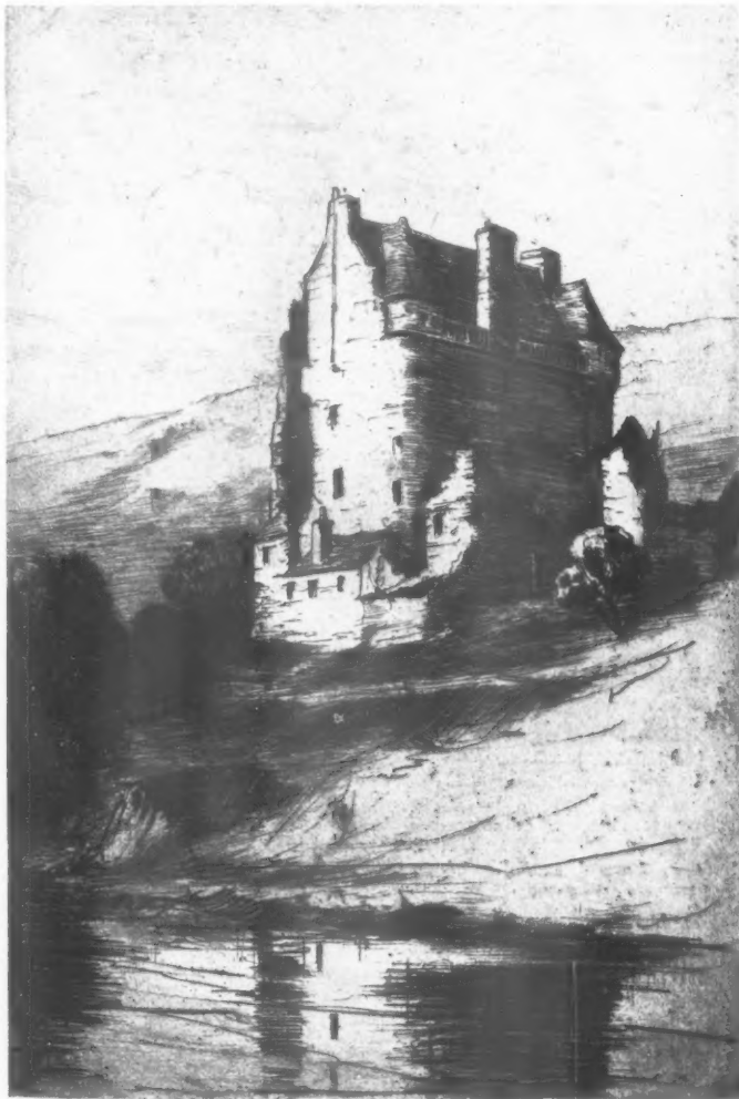
Fig. 2.—NEIDPATH CASTLE, PEEBLES SHIRE.
