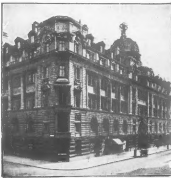
Electro House. Covered with Patent Vulcanite Roofing.
