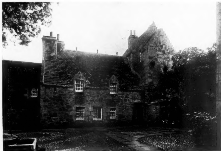
Fig. 9.—SOUTH SIDE OF COURTYARD.
