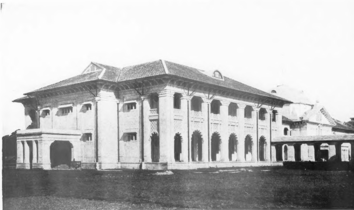
MAIN BUILDING FROM SOUTH-EAST.
