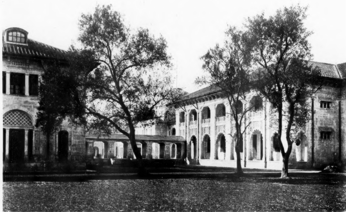
VIEW BETWEEN BAR CHAMBERS AND MAIN BUILDING.
