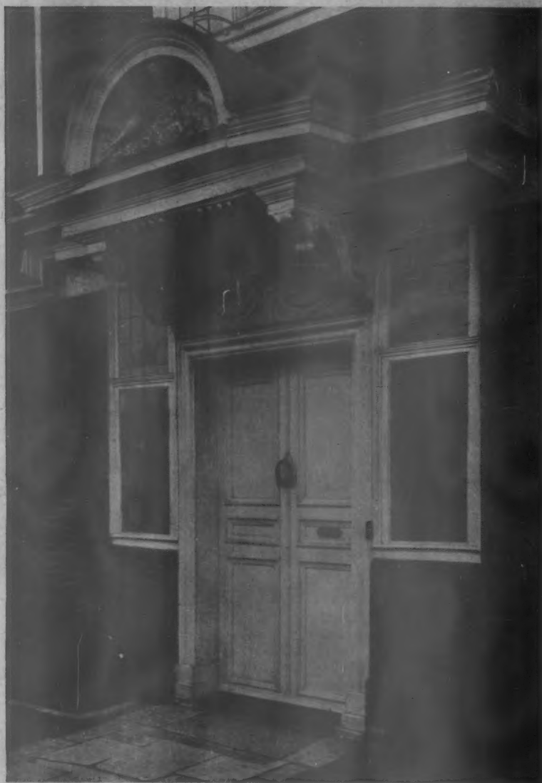
Doorway and Hood, Rampyndene, Burwash, Sussex.
