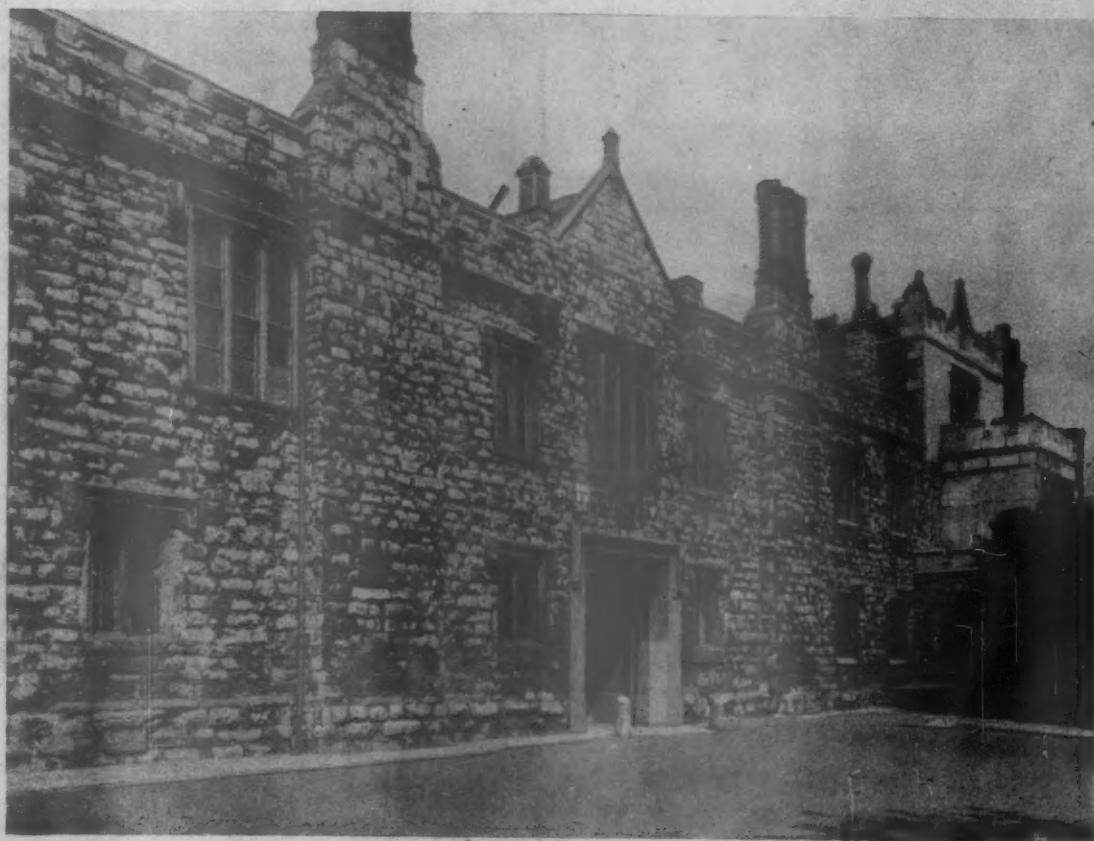
South Front of Master's Lodge (Howard House), 1543-71.
