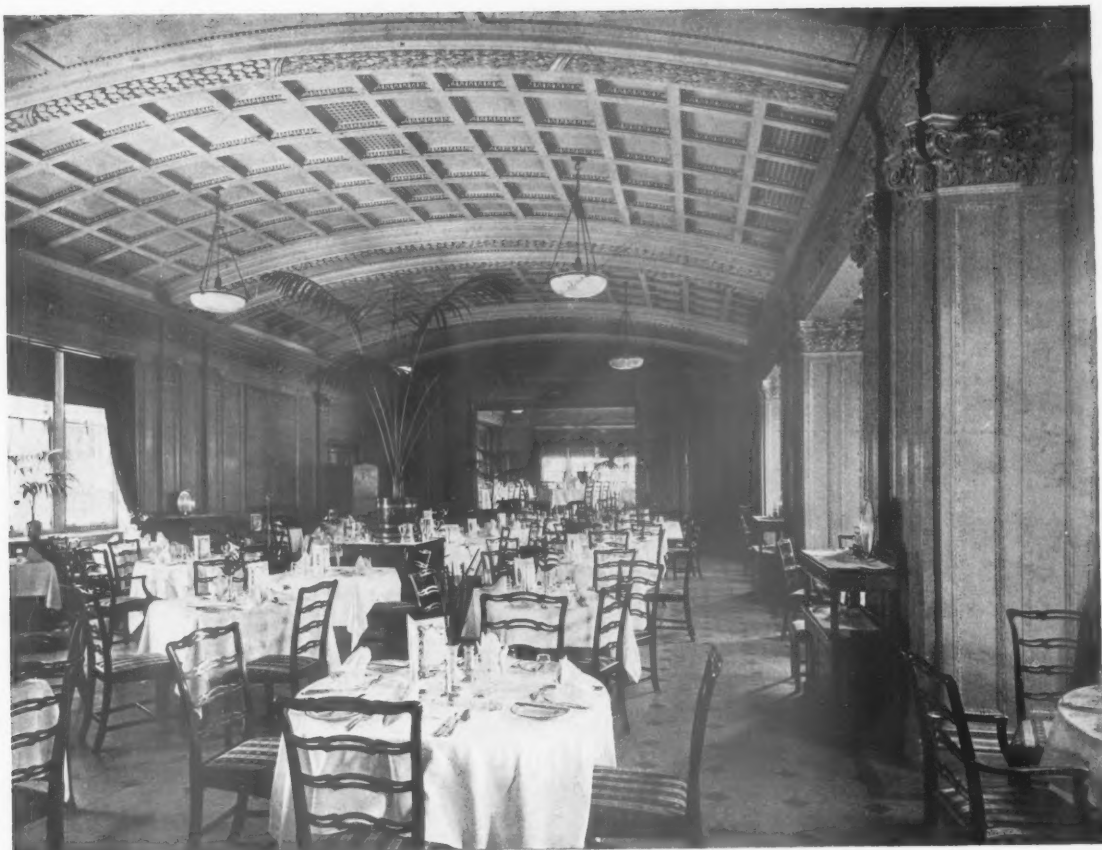
Restaurant, looking towards Annexe.
