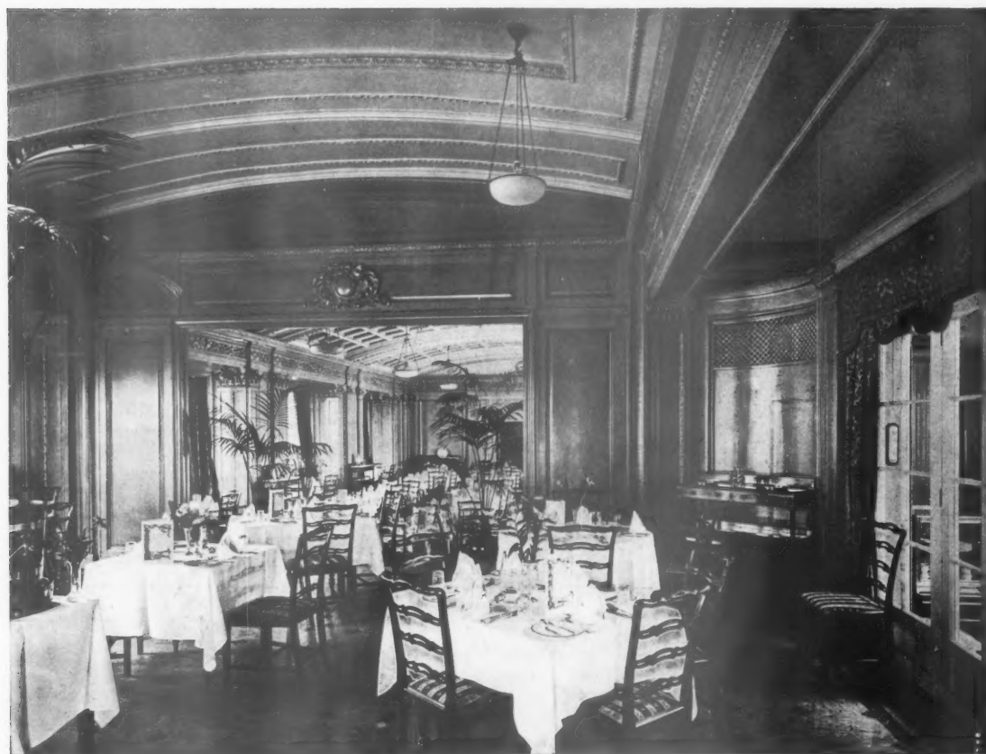
Annexe, looking into Restaurant.
