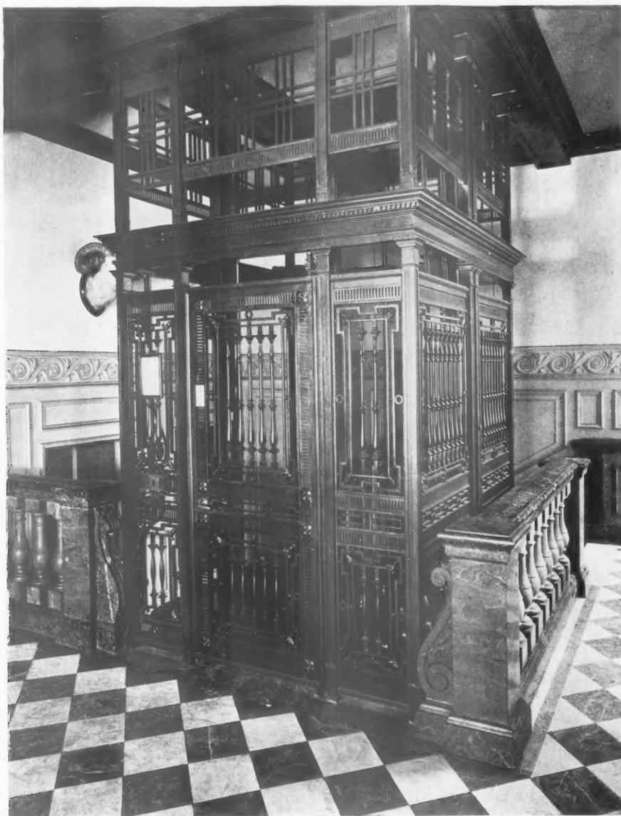
LIFT ENCLOSURE, FIRST FLOOR.
