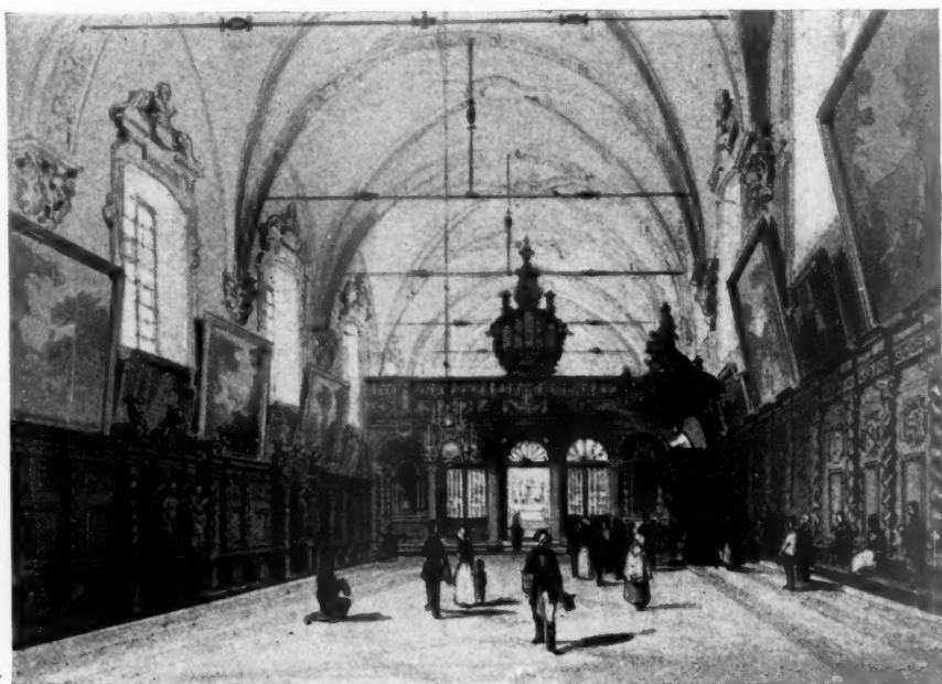
INTERIOR OF THE CHURCH OF ST. ANNE.
