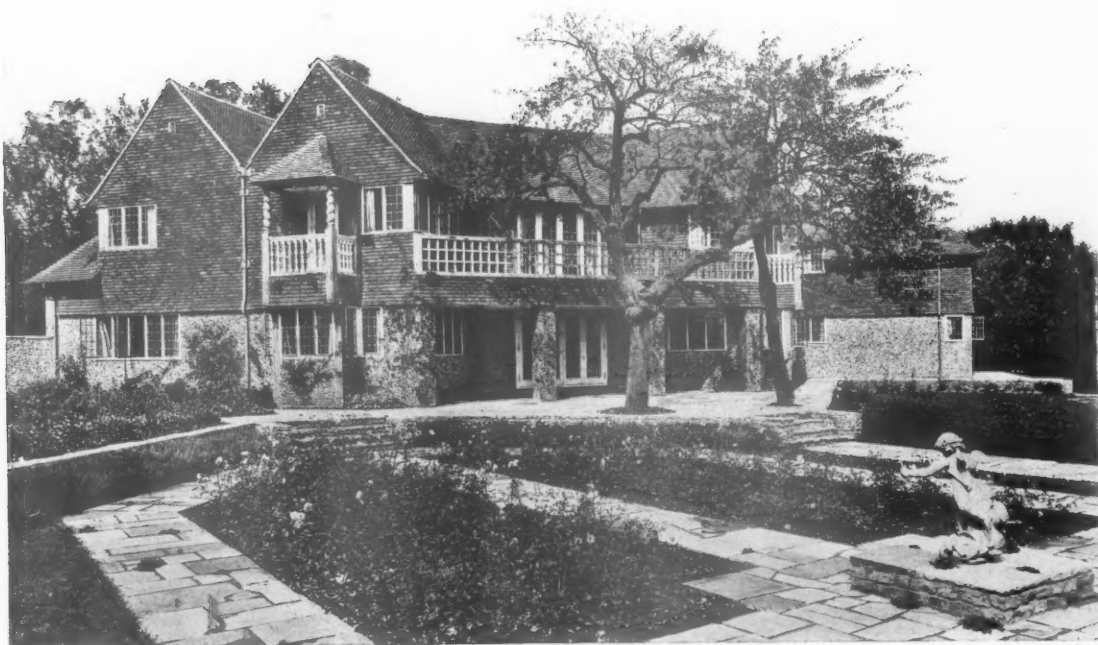
View towards the South-west.
