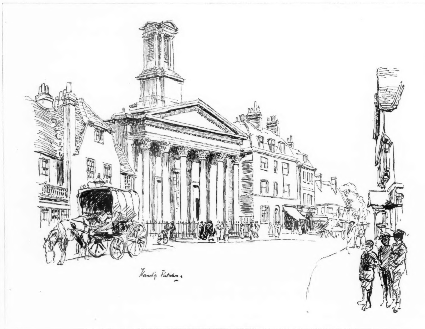
THE BEAR INN AND ST. MARY'S CHAPEL, CASTLE STREET.
