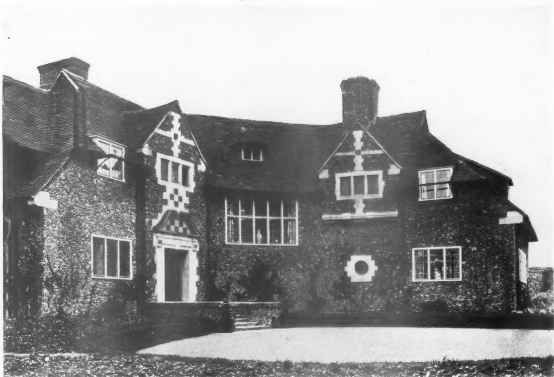
View of Entrance Front.
