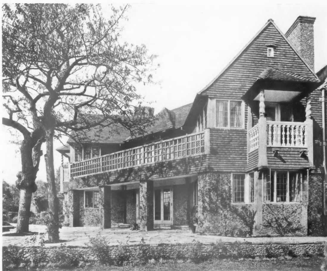
View towards the South-west.
