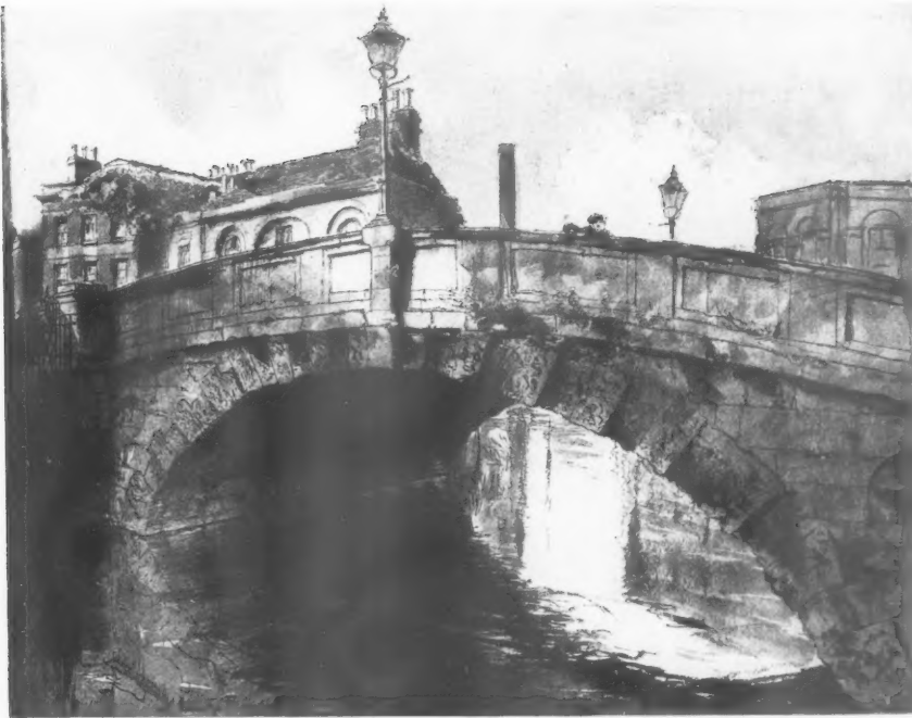
STONE BRIDGE OVER THE RIVER KENNET.
