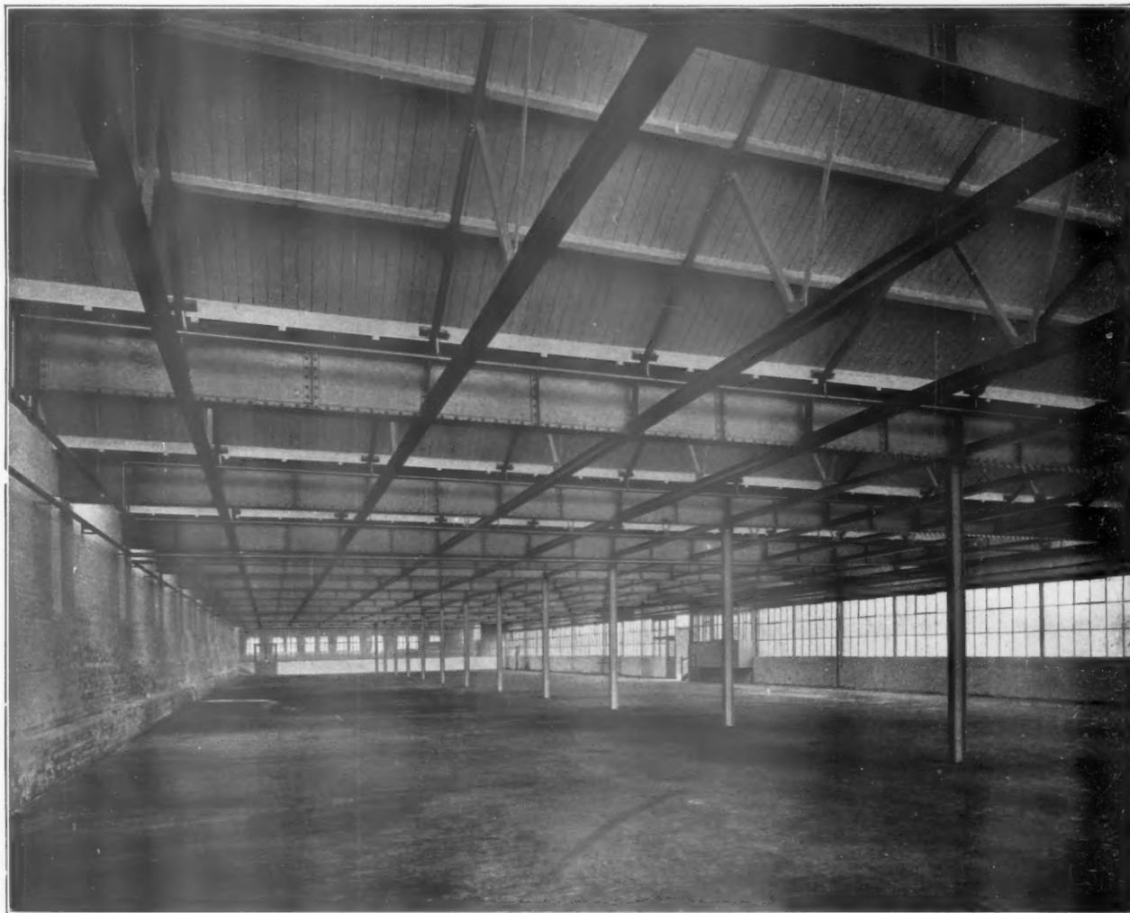
Example of Modern Factory Construction.
