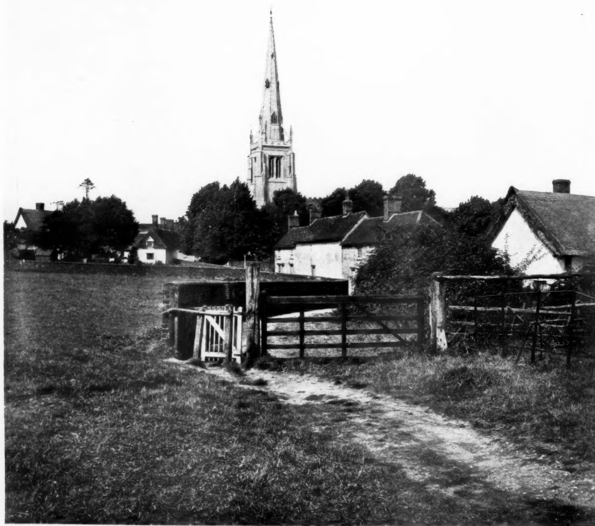
THE BYPATH ENTRANCE THROUGH THE MILL FIELD.
