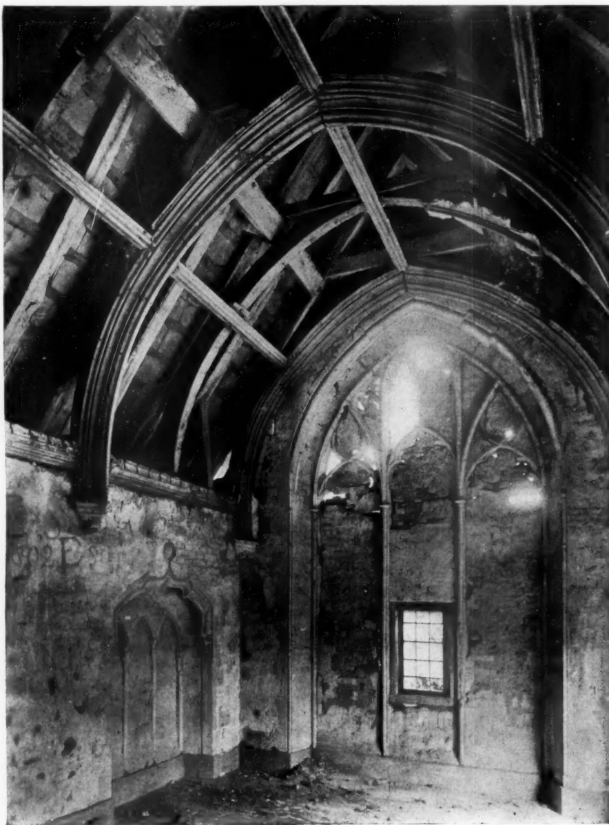
INTERIOR, LOOKING EAST.
