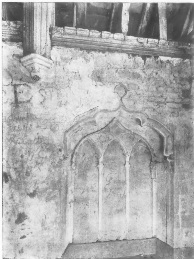
DETAIL OF INTERIOR (NORTH WALL).
