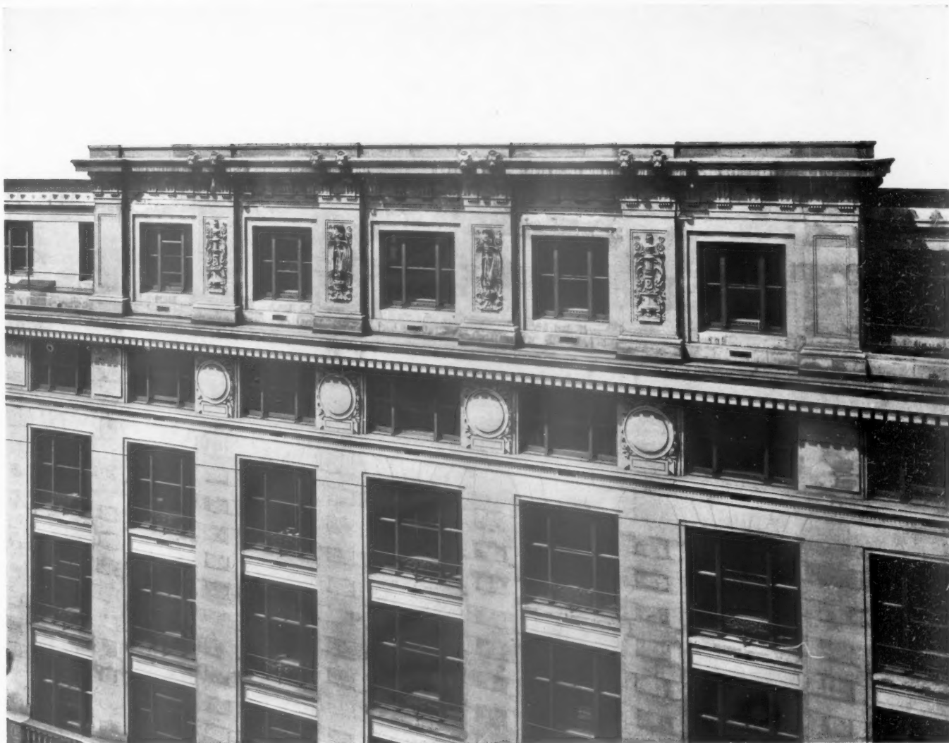
View of Upper Storeys and Attic.
