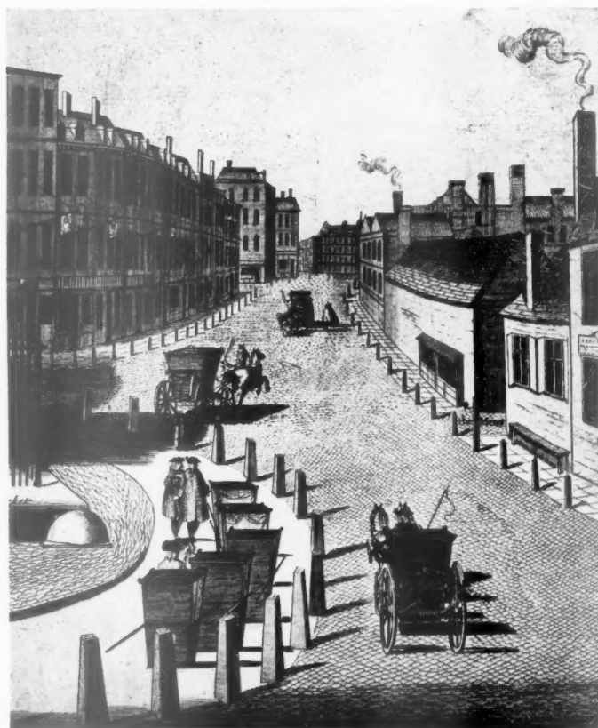
A VIEW OF CHARING CROSS, 1737, SHOWING ENTRANCE TO THE MEWS.
