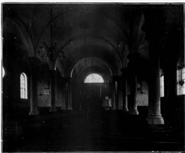
COLDSTREAM PARISH CHURCH. EXPANDED METAL LATHING AND PLASTER CEILINGS. ARCHITECT: Mr. J. M. DICK PEDDIE, M.S.A., EDINBURGH.
