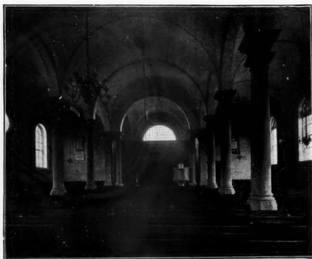
COLDSTREAM PARISH CHURCH. EXPANDED METAL LATHING AND PLASTER CEILINGS. ARCHITECT: MR. J. M. DIC & PEDDIE, M.S.A., EDINBURGH.
