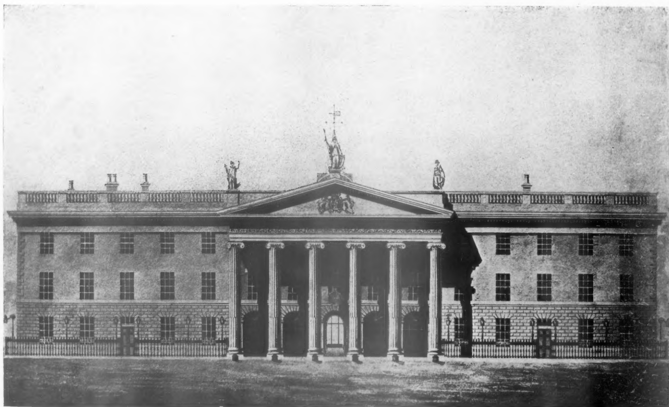
THE FAÇADE OF THE GENERAL POST OFFICE, DUBLIN, AS IT APPEARED ABOUT 1820.
