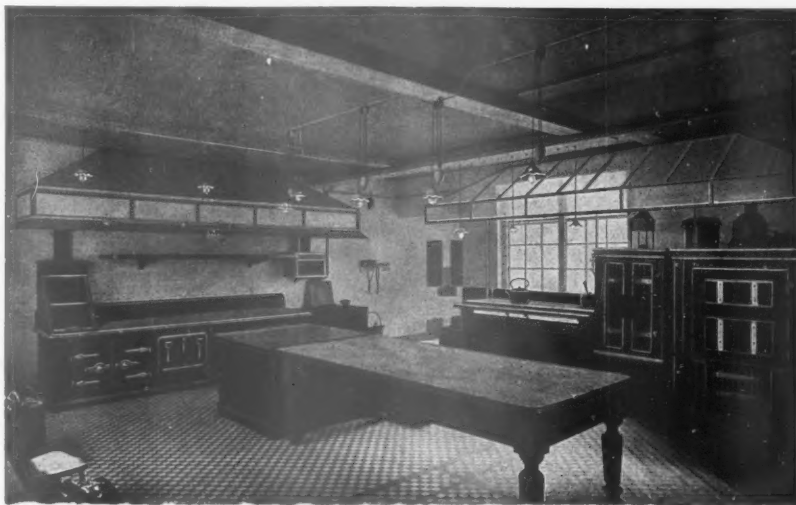
The Kitchen of 46, Grosvenor Street, W., showing Coal Range (French pattern), with Charcoal Grill, Plate Rack and Tiled Hood; Gas Hot Plate with Ovens under, Gas Roasting Oven, Gas Pastry Oven, central Wood Table with Steam Hot Closet at one end; Glazed Hood over Gas Fittings. Architects: Messrs. Detmar Blow and Fernand Billerey.
