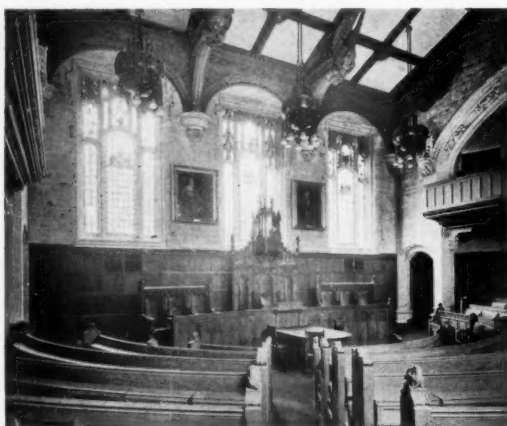
MIDDLESEX GUILDHALL. Architects, Messrs. Gibson, Skipworth & Gordon.
