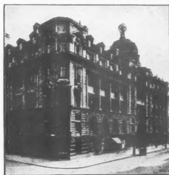
Electra House. Covered with Patent Vulcanite Roofing.
