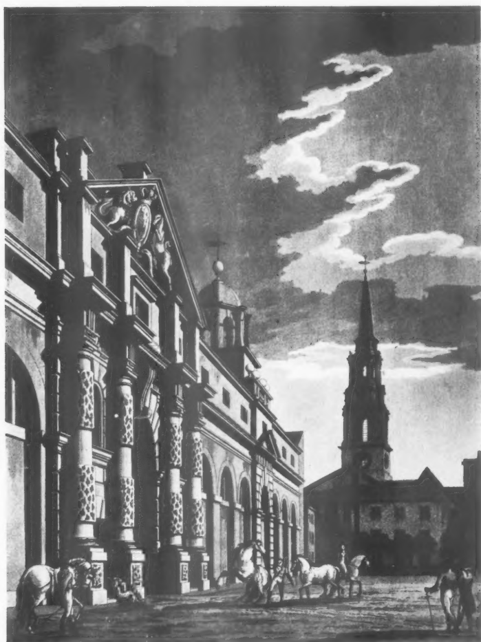
EXTERIOR OF THE MEWS, 1794.
