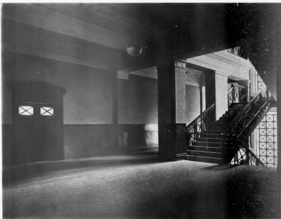
STAIRCASE AND LANDING, UPPER GROUND FLOOR.
