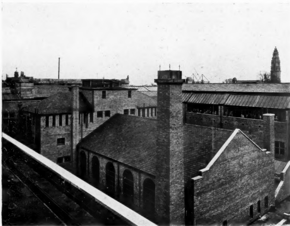
REAR VIEW FROM ROOF LEVEL.
