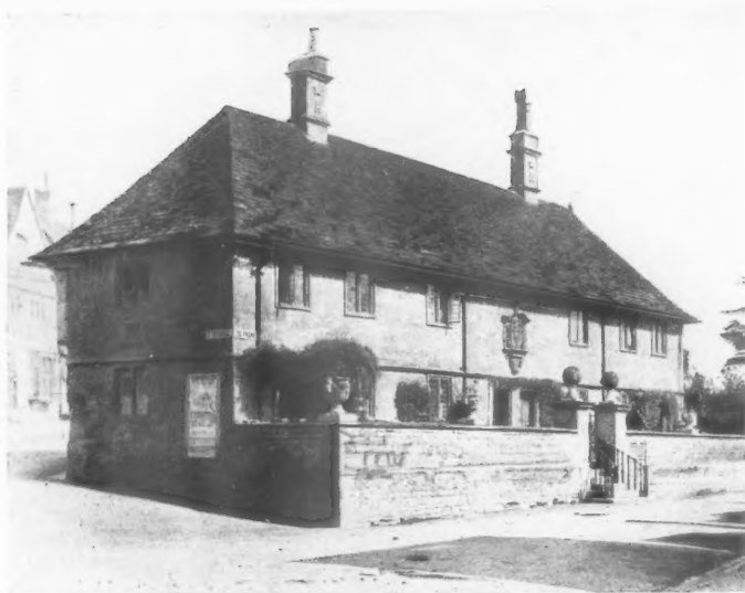
HALL'S ALMSHOUSES, BRADFORD-ON-AVON.
