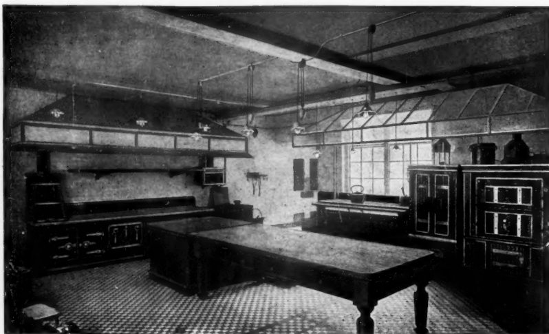
The Kitchen of a Private Mansion, showing Coal Wall Hot Plate, Charcoal Grill, Gas Grill, Gas Hot Plate with Ovens, Large Gas Roasting Oven, Gas Pastry Oven, and Steam Heated Hot Closet (in centre of kitchen), also Tiled and Glass Ventilation Hoods.
