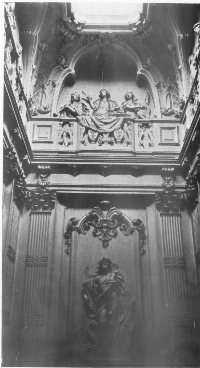
PLASTERWORK IN STAIRCASE HALL.
