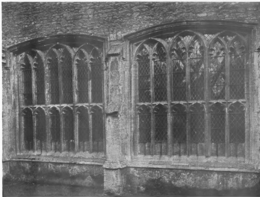
WINDOWS IN NORTH AISLE, FARINGDON CHURCH: EXTERIOR.
