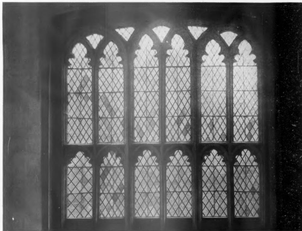
WINDOWS IN NORTH AISLE, FARINGDON CHURCH: INTERIOR.
