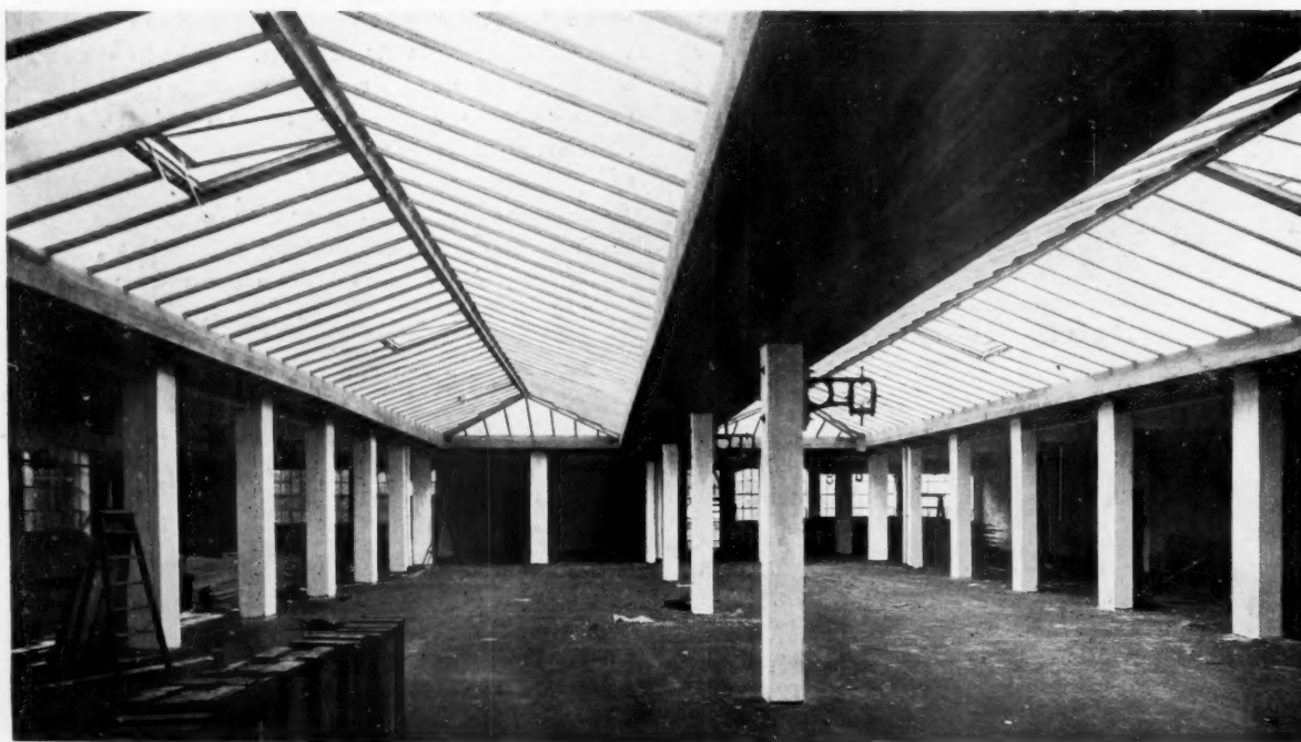
LANTERN LIGHTS, MESSRS. EDWARDS' FACTORY, NORWICH (INTERIOR). CONSTRUCTED WITHOUT PRINCIPALS.
