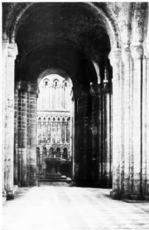
END OF SOUTH AISLE OF NAVE
