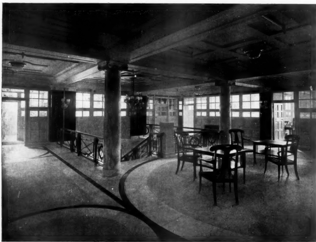
THE KODAK BUILDING, KINGSWAY: RECEPTION HALL, FIRST FLOOR J. J. BURNET, ARCHITECT
