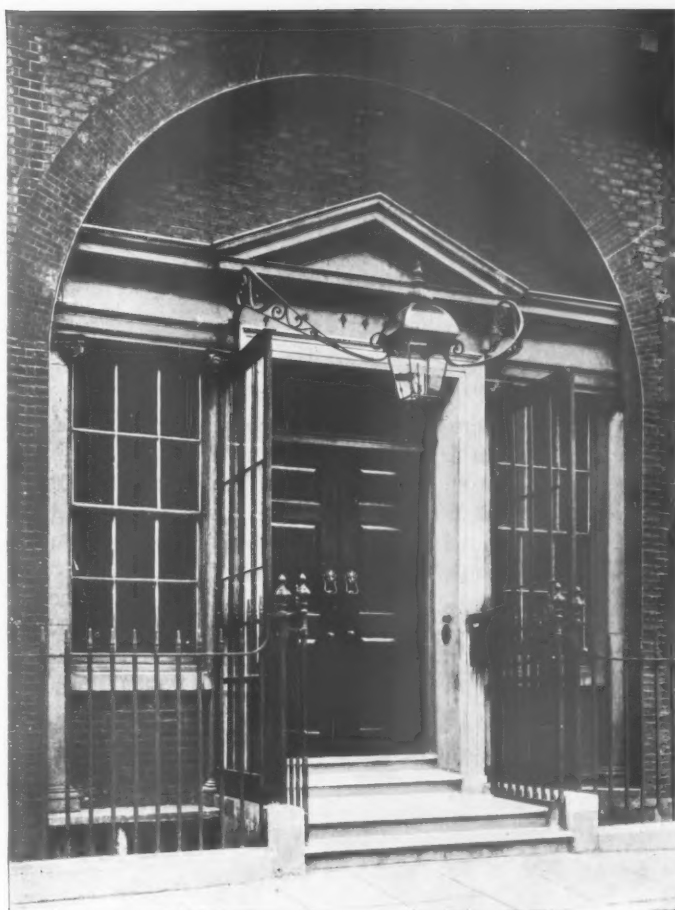
NO. 1 STRATTON STREET, LONDON (1790), BY BRETTINGHAM (From "London Houses," by Richardson and Gill)
