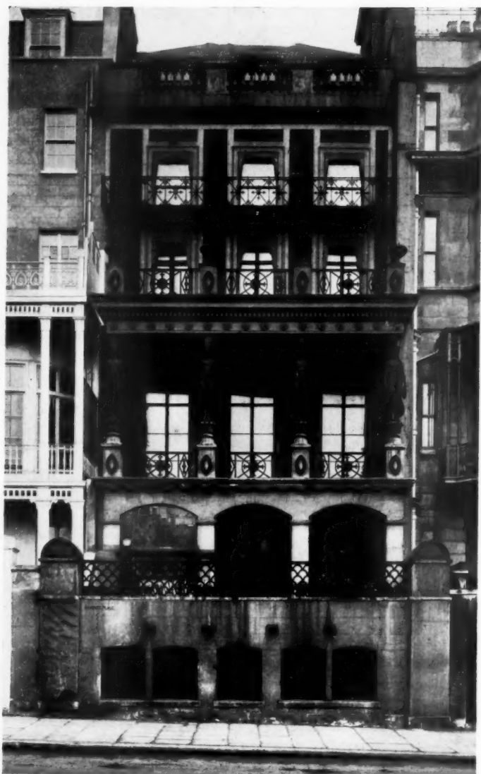
NO. 3 SEAMORE PLACE, PARK LANE, LONDON, W. (LATELY DEMOLISHED). JOHN PAPWORTH, ARCHITECT (From a photograph lent by Mr. B. T. Batsford)
