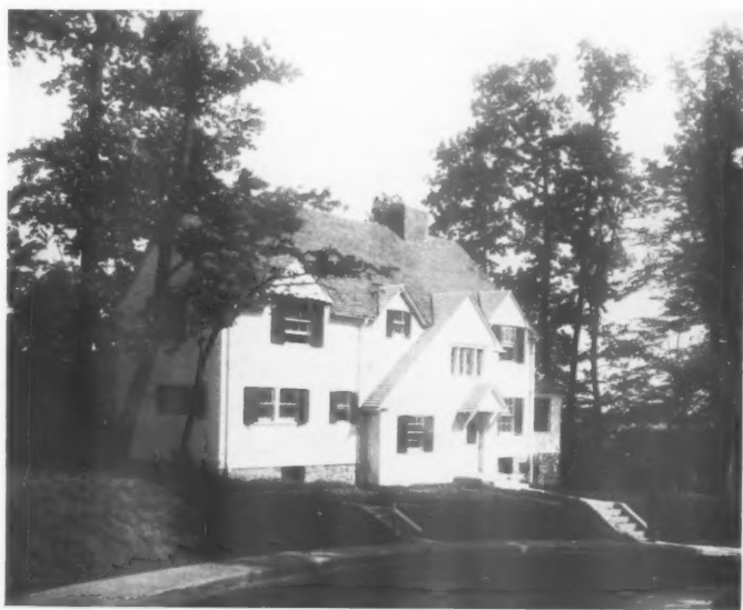
COTTAGE ON MERRYMOUNT ROAD, ROLAND PARK, BALTIMORE
