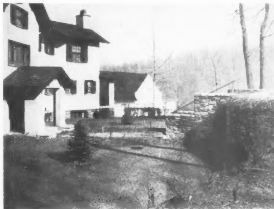
VIEW OF HOUSE SHOWING SUNKEN GARDEN AND WALL
