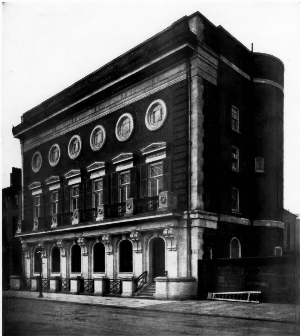
THE STUDENTS' UNION, LIVERPOOL: FAÇADE TO BEDFORD STREET PROFESSOR C. H. REILLY, M.A., A.R.I.B.A., ARCHITECT
