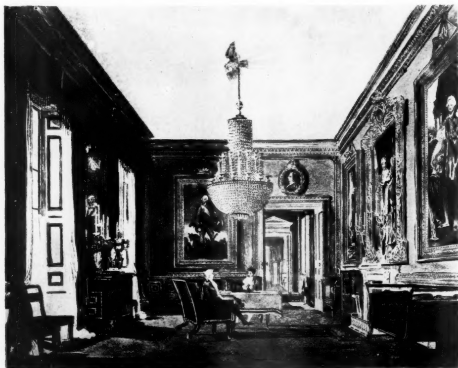
THE WEST ANTE-ROOM, CARLTON HOUSE
