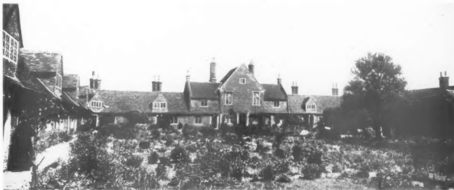
EAST ELEVATION TO QUADRANGLE
