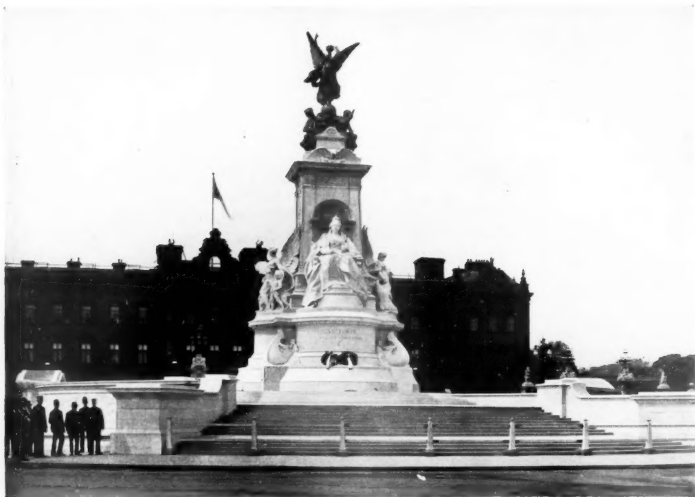
GENERAL VIEW FROM SOUTH-EAST
