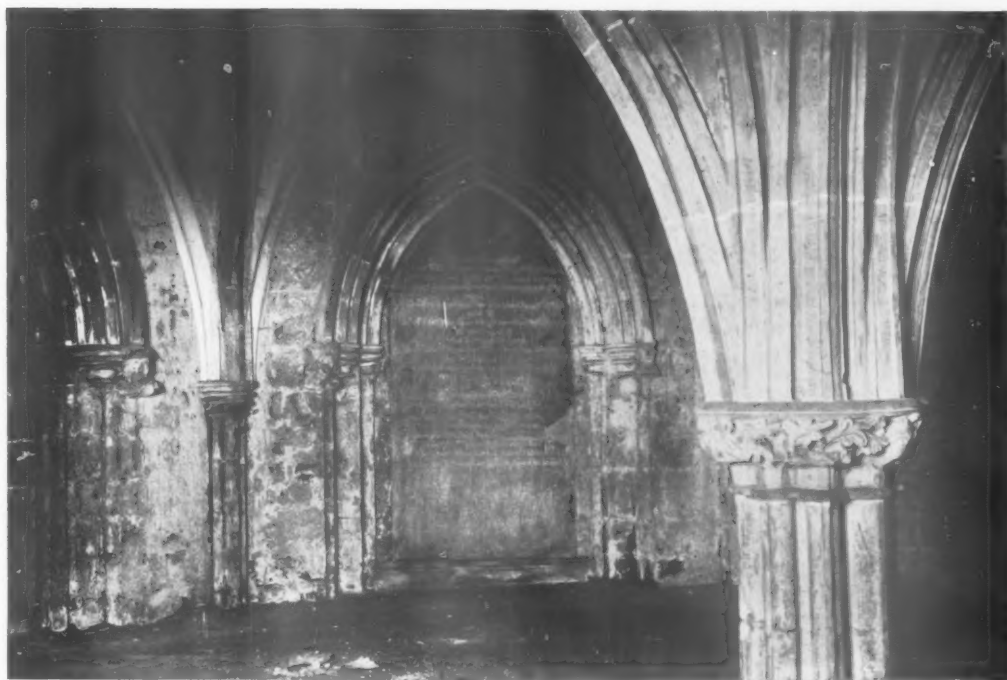
INTERIOR, LOOKING NORTH-WEST
