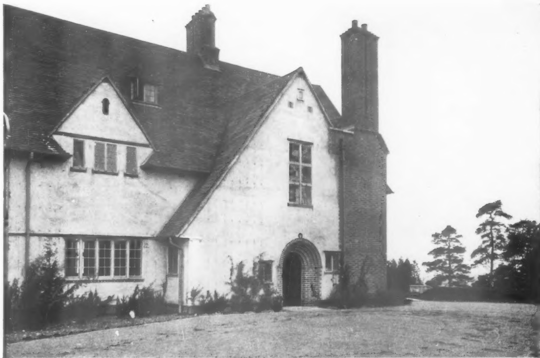
North front, with entrance doorway.
