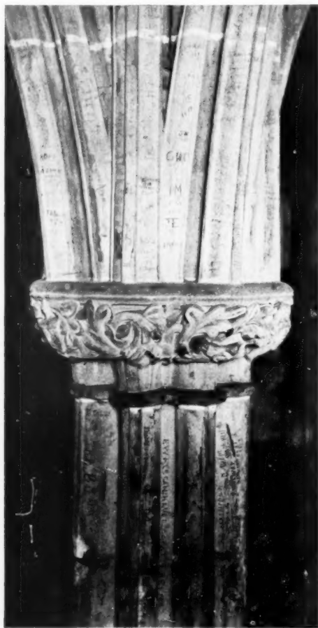
CENTRAL PIER, WITH CAPITALS, COCKERSAND CHAPTER-HOUSE
