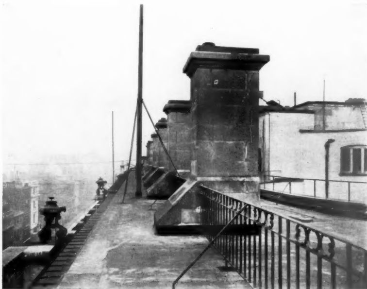
VIEW ON ROOF, SHOWING SET-BACK OF CHIMNEYS
