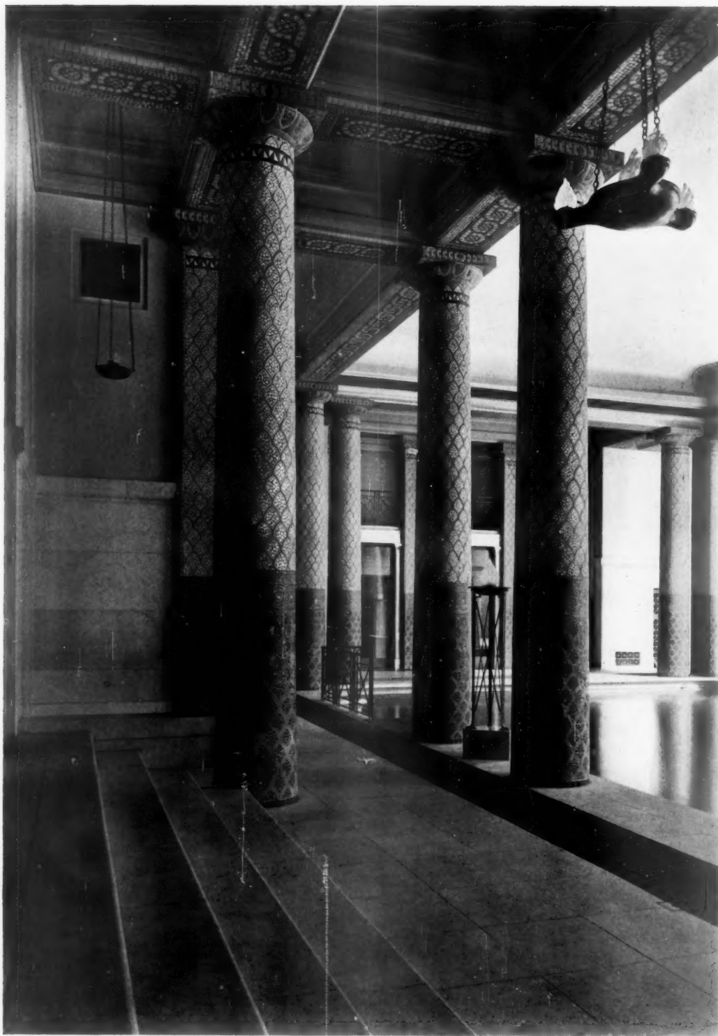
DETAIL VIEW OF COLUMNS, IN SWIMMING-BATH
