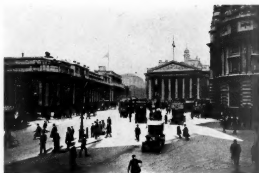
TRAFFIC CENTRE IN FRONT OF THE MANSION HOUSE, LONDON
