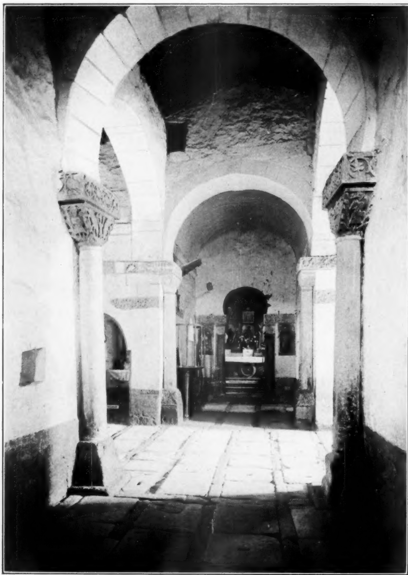
INTERIOR VIEW OF SAN PEDRO DE LA NAVE.
