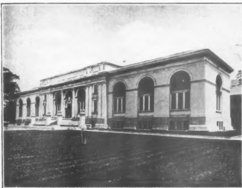
LIBRARY, COLUMBUS, OHIO. ALBERT RANDOLPH ROSS, ARCHITECT.
