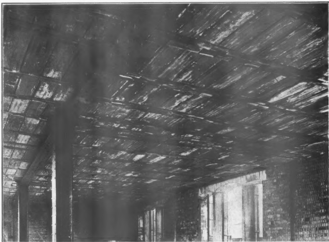
VIEW SHOWING THE FLOOR CONSTRUCTION ON THE FRAZZI SYSTEM.
