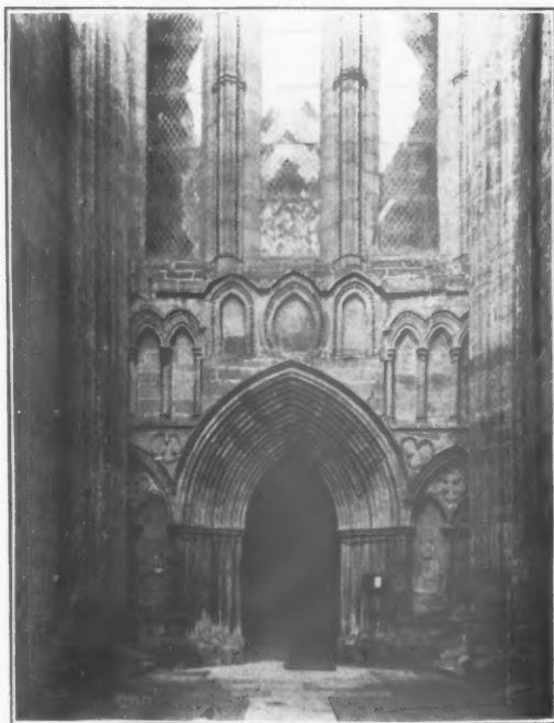
WEST FRONT OF THE NAVE.
