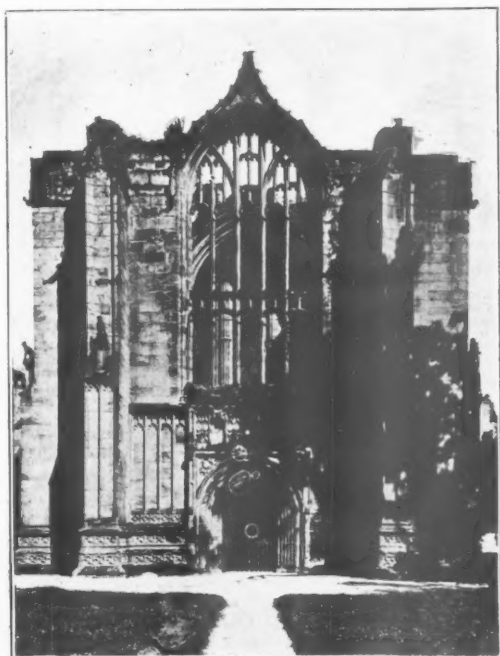
WEST FRONT OF THE TOWER.
