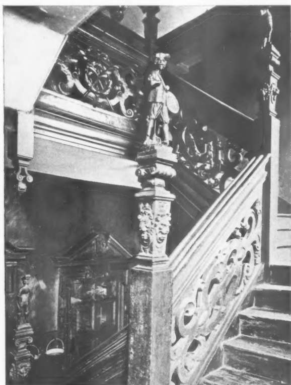
STAIRCASE, CROMWELL HOUSE, HIGHGATE.
