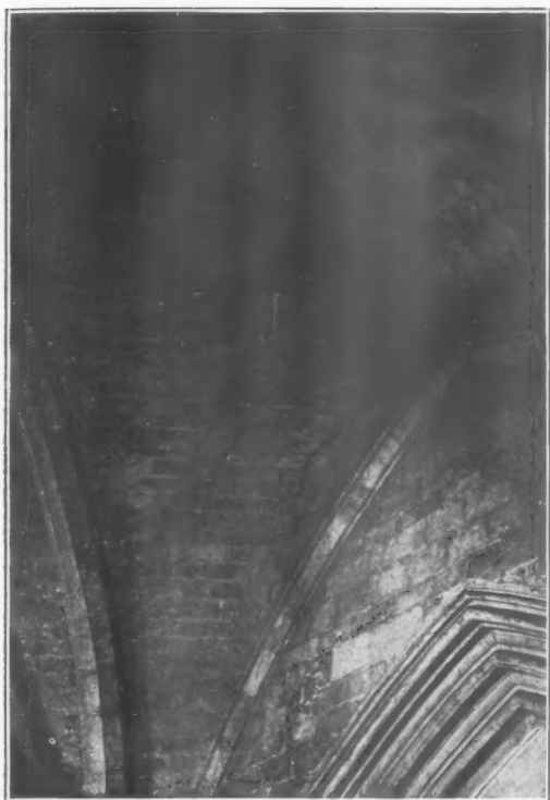
CENTRE BAY TO CENIRE VAULT, PRESBYTERY, LOOKING SOUTH-EAST.
