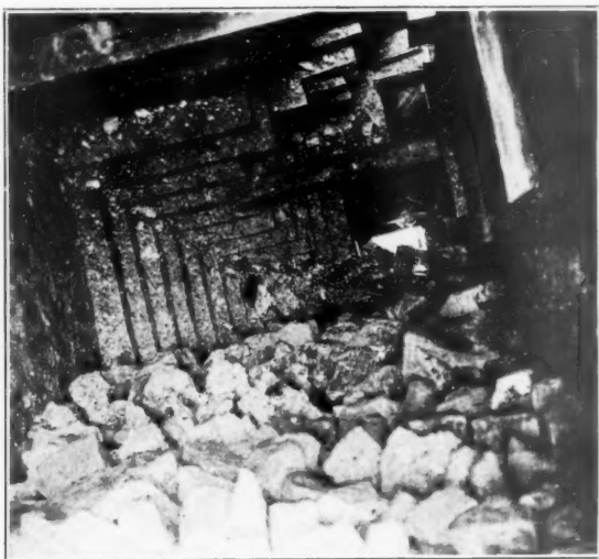
SHOWING NEW BRICK FOOTINGS TO THE WALLS
