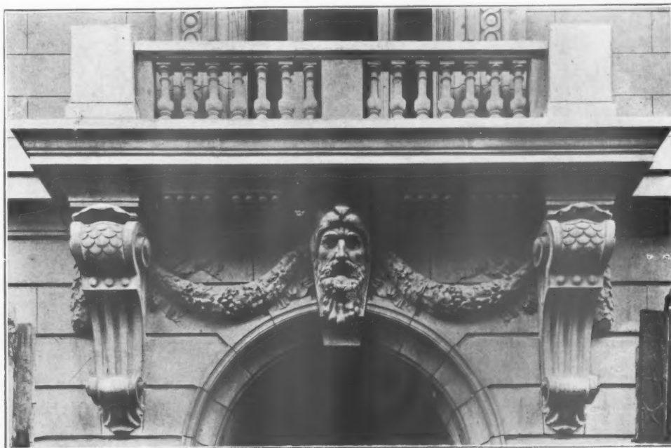
DETAIL OVER DOOR IN ALDWYCH.
