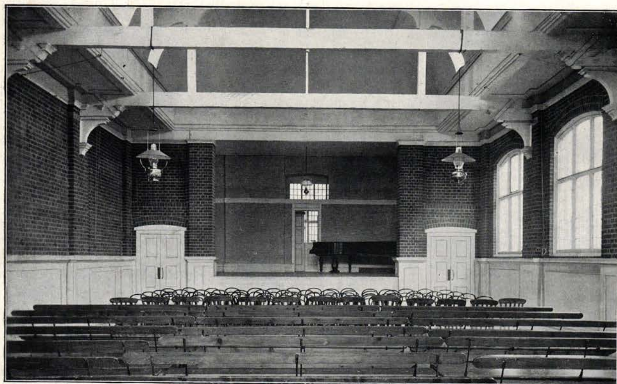
ORFORD TOWN HALL, SUFFOLK. HARKY SIRR AND E. J. ROPE, ARCHITECTS.
