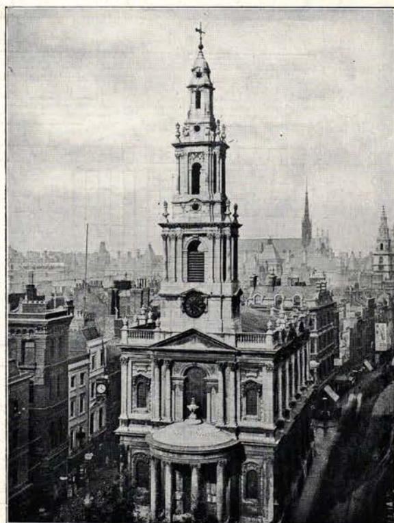
ST. MARY-LE-STRAND, LONDON. JAMES GIBBS, ARCHITECT.
