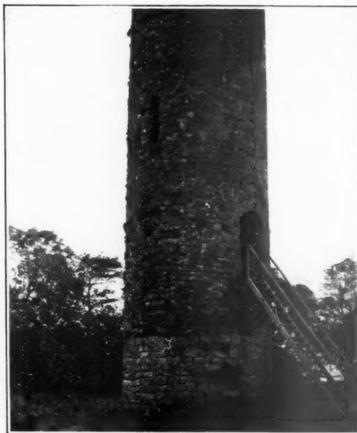
ROUND TOWER, KILDARE, SHOWING VARIETY OF MASONRY.
