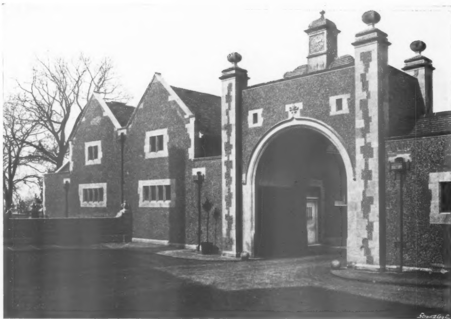
Archway from Courtyard to Stable.
