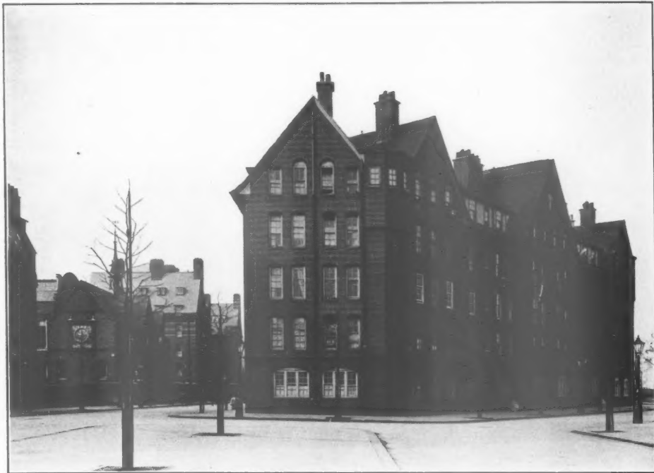
TURNER BUILDINGS, HERRICK STREET, MILBANK
