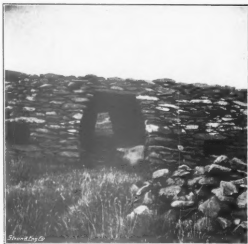
DUNBEG. FROM INSIDE, ENTRANCE AND GUARD-ROOMS.
