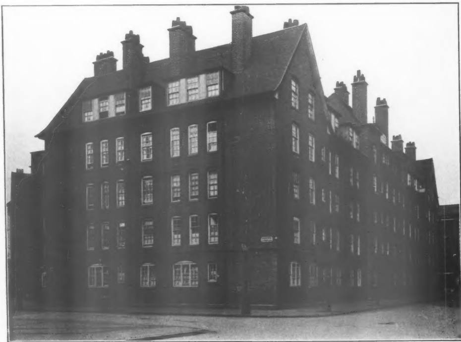
LAWRENCE BUILDINGS, HERRICK STREET, MILBANK.
