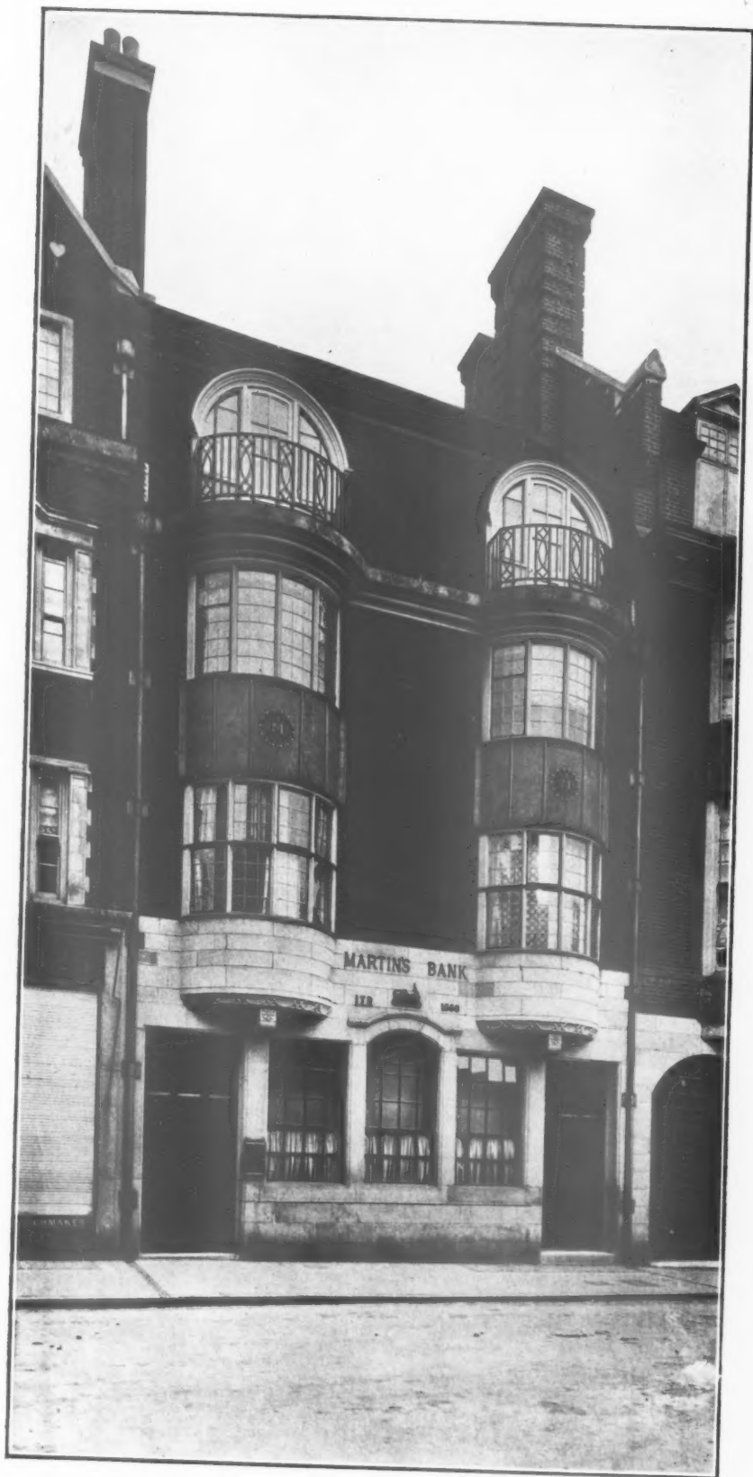
BANK PREMISES, BROMLEY. ERNEST NEWTON, ARCHITECT.
