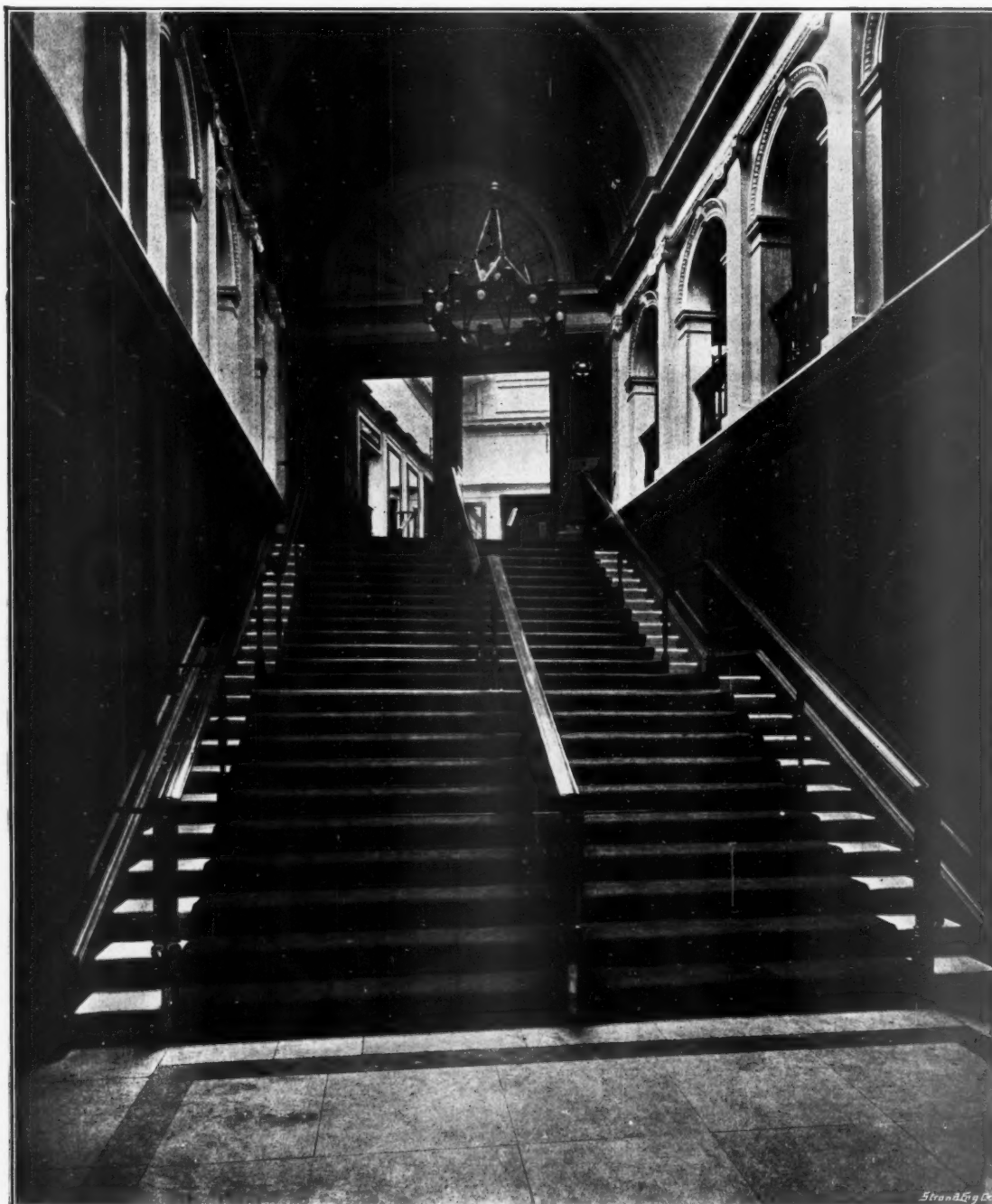
135, 136, 137, NEW BOND STREET, LONDON. THE STAIRCASE. WALTER CAVE, ARCHITECT.
