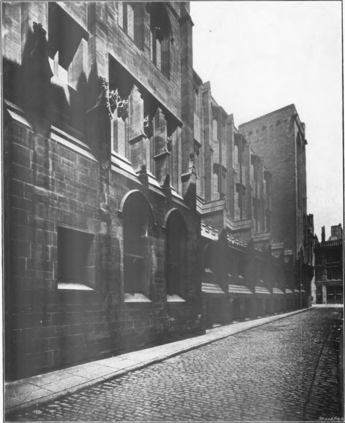
THE RYLANDS MEMORIAL LIBRARY, MANCHESTER. ELEVATION TO SPINNINGFIELD. BASIL CHAMPNEYS, ARCHITECT.
