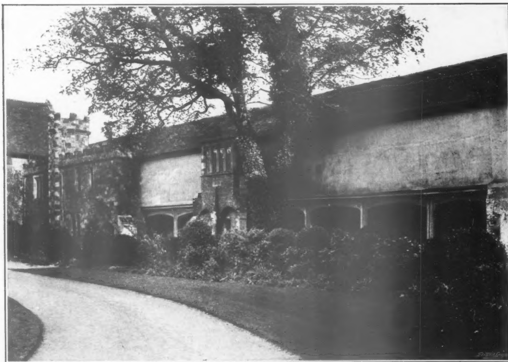
THE AMBULATORY, AND INFIRMARY OVER, FROM THE SOUTH-WEST.
