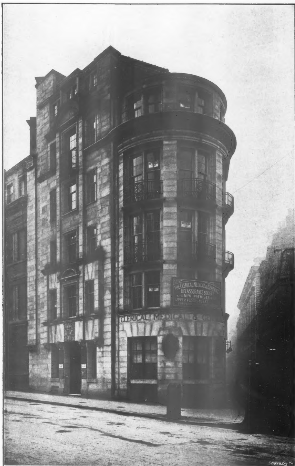
CLERICAL, MEDICAL, AND GENERAL ASSURANCE CO.'S NEW BRANCH OFFICE, KING WILLIAM STREET, LONDON, E.C. W. DUNN AND R. WATSON, ARCHITECTS.
