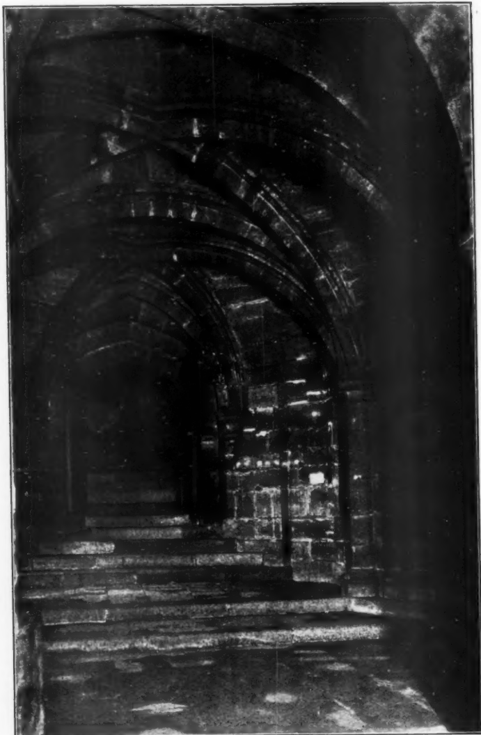
SOUTH-WEST COMPARTMENT, LOOKING WEST.
