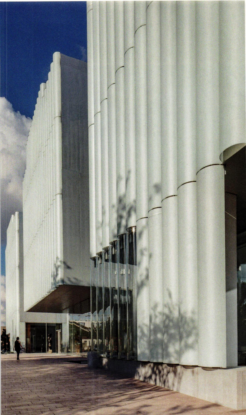
CLAD IN half-tubes of etched glass (left), the translucent facade is punctuated by a section of clear curved glazing near an entrance (above).
