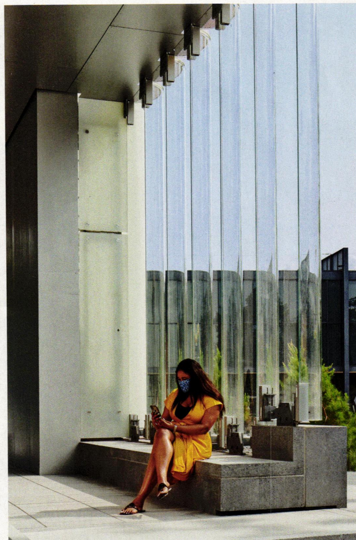
CLAD IN half-tubes of etched glass (left), the translucent facade is punctuated by a section of clear curved glazing near an entrance (above).
