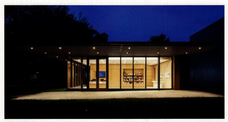
Part solid and part trelliswork, the large cantilevered roof of the steel-frame Welcome House allows groups of visitors to congregate outdoors, protected from the elements, before entering the chapel.
