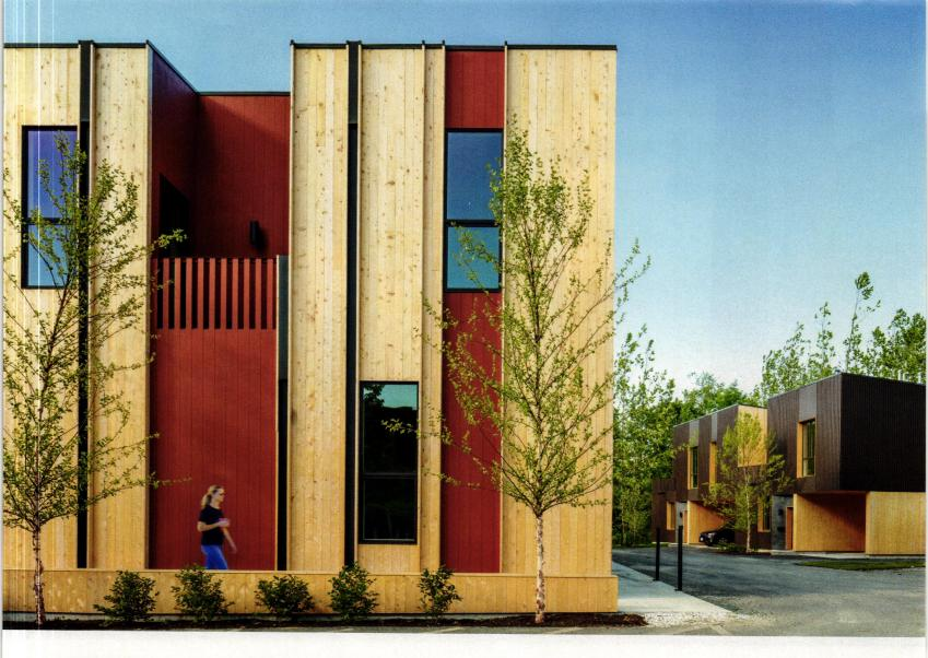
MODERN MILL is a second component of the condominium apartments at Cable Mills. Here terra-cotta-colored fly ash and polymer panels alternate with Alaskan yellow cedar (above). In River Houses, two views of a duplex living area (opposite) demonstrate how the atrium brings light into the living and dining spaces.
