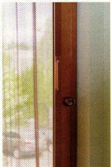
Copper-clad wire fabric is naturally antimicrobial and can be used to divide spaces or provide solar and shade control.
