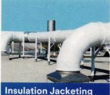
Our tough, long lasting laminates provide mechanical duct and pipe protection on roofs or other exposed areas to prevent moisture from migrating into insulation, even at seams.
