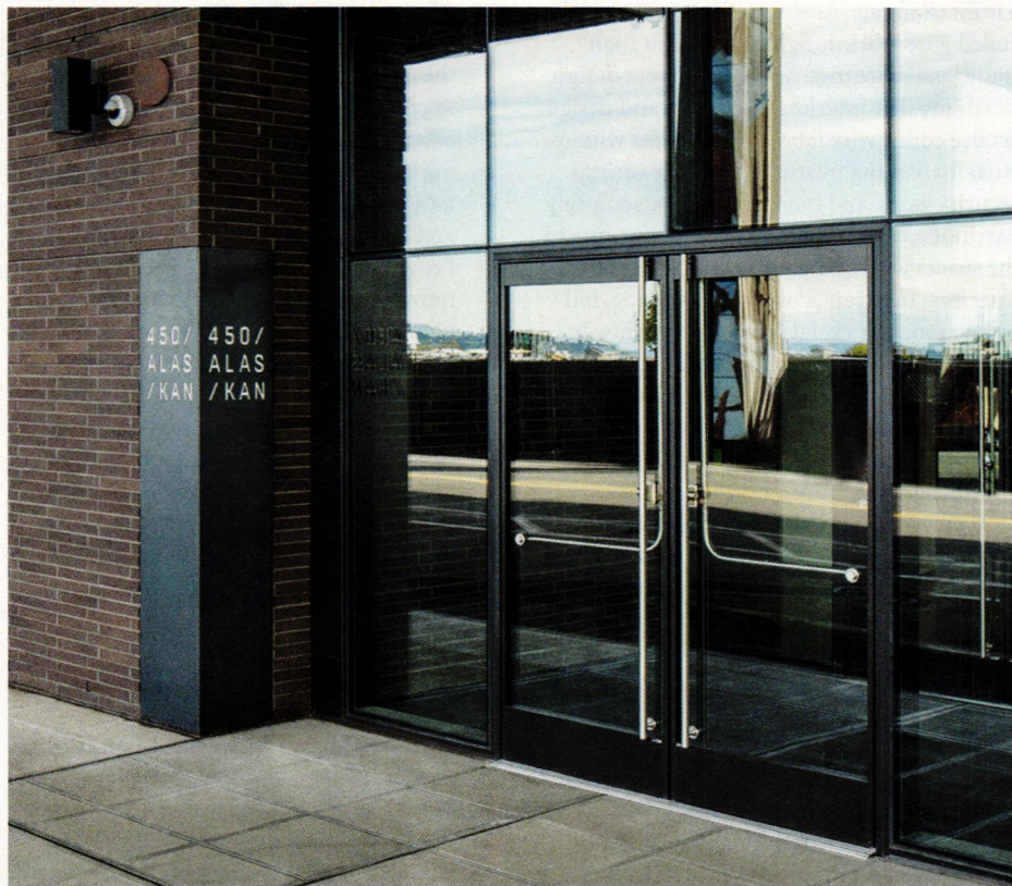
High-performance entrance systems provide greater resilience through properly specified components and enhanced thermal properties, all while offering an elegant design using ultra-narrow door stiles.
