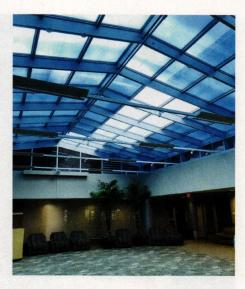
Dynamic glazing offers a new option for shading in buildings, but it is expensive and difficult for retrofit applications.
