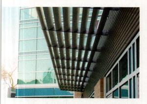
Fixed exterior shading creates an often striking but non-flexible solar shading option for buildings.
