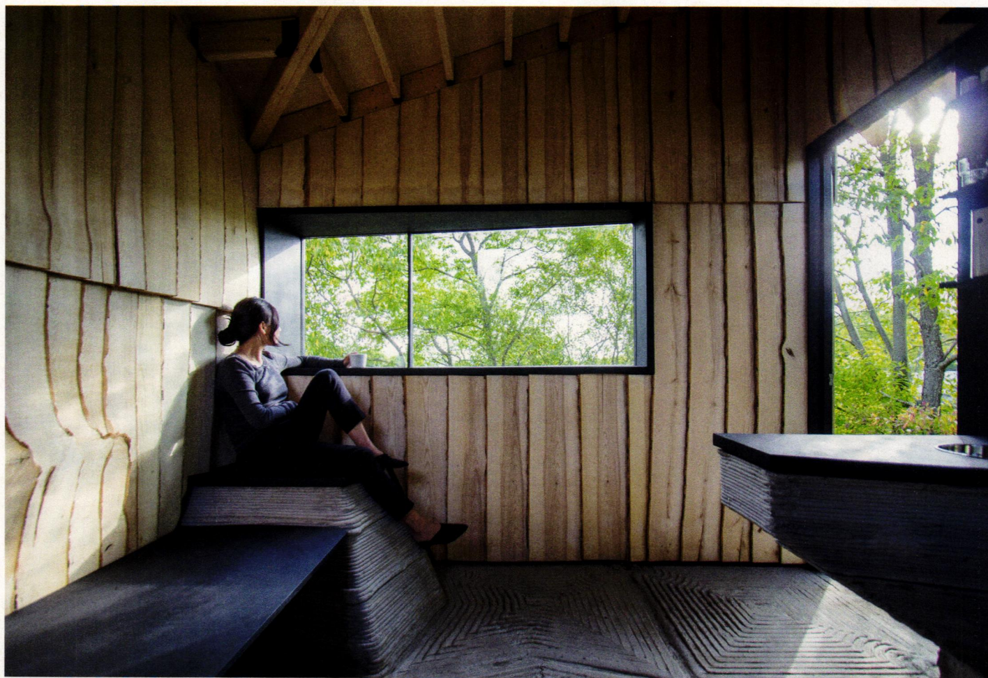
3-D LASER SCANNING and robotics-based manufacturing techniques helped HANNAH Architecture and Design create the 100-square-foot Ashen Cabin (opposite and above) in upstate New York from trees killed by the emerald ash borer.
