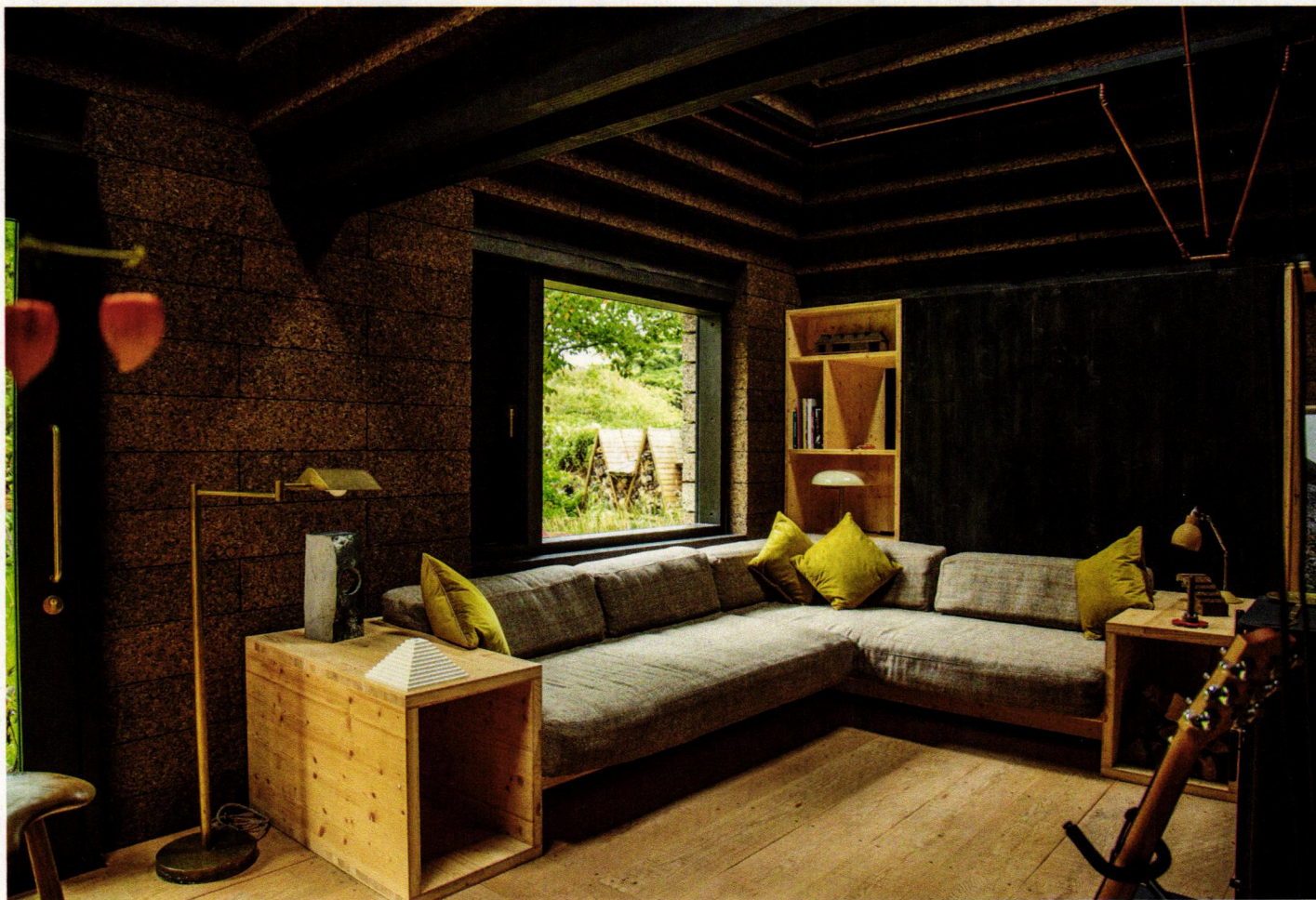
THE STRUCTURE , weather envelope, insulation, and interior finish (above) of the Cork House consist almost entirely of cork blocks (left) that are tongue-and-groove friction-fit together.
