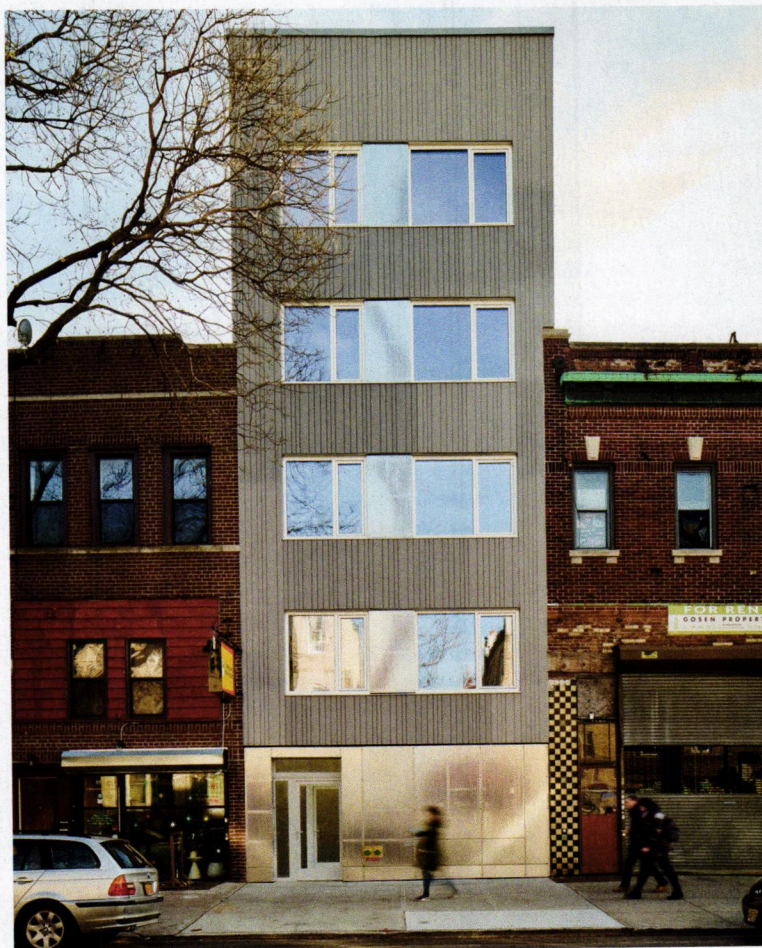
A five-story condo building in Brooklyn (left) and a 55-unit rental apartment tower in Manhattan (bottom), both recently completed and designed by ZH Architects, deploy such features as highly insulated and airtight facades, triple-glazed windows, and minimized thermal bridges. Both are expected to meet Local Law 97's anticipated emissions limits for 2050.
