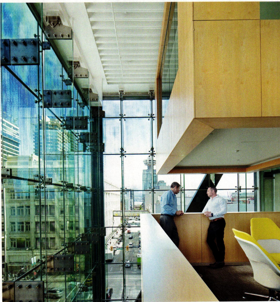
Long-span composite floors blend in with the rest of the building construction and can create a finished ceiling appearance in addition to providing a strong, economical floor structure option.
