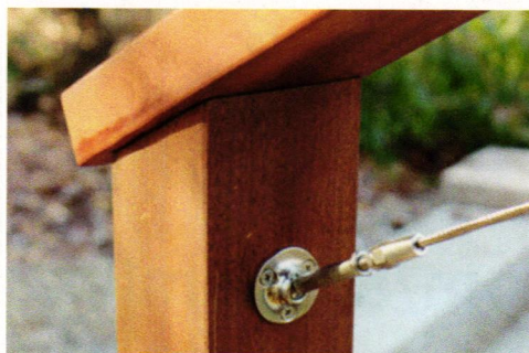
The two common types of cable railing systems include surface-mount systems (left) and through-post systems (center). Note that through-post systems will require some staggering of cable heights at corners (right).
