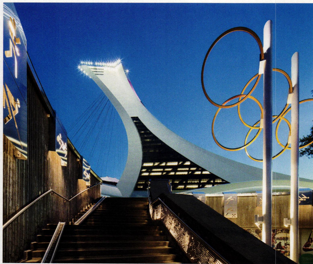
The Olympic stadium's retractable Kevlar roof is supported by cables that hang from a futuristic, swooping tower. The 541-foot-tall structure now houses corporate offices on its unique triangular floor plates, which get smaller as they rise.
