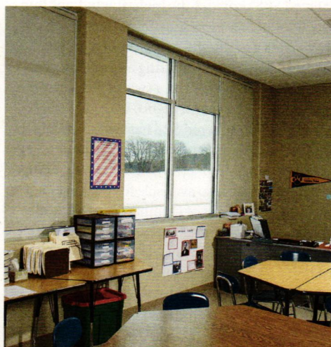
Interior cordless window shades with textured fabric can provide privacy or maintain connections to the exterior while helping with energy performance by reducing solar heat gain.
