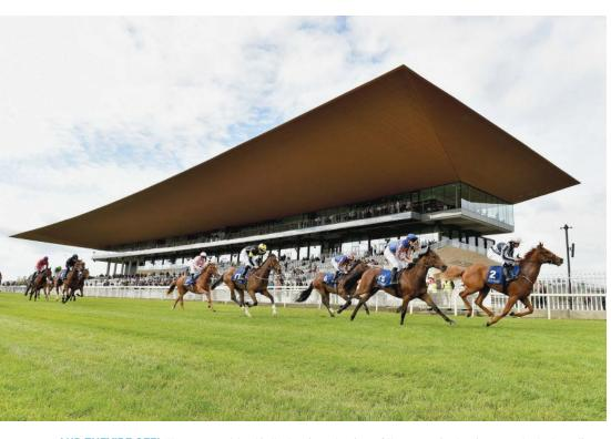
**AND THEY'RE OFF!** The new grandstand is the heroic centerpiece of the reorganized racing grounds. Its dramatic cantilevered roof is clad in perforated copper-colored aluminum panels.
