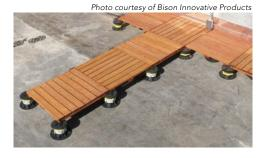
Shown here is an installation of a pedestal deck system supporting ipê wood tiles on a rooftop deck.
