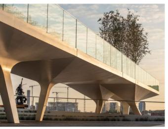
Twenty-eight structural columns support the first phase of the Tide, which opened July 5.
