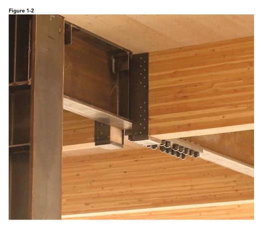
At the Hawker Architects-designed First Tech Credit Union in Palo Alto, California, a crosslaminated timber (CLT) floor is supported by a glue-laminated timber structure.
