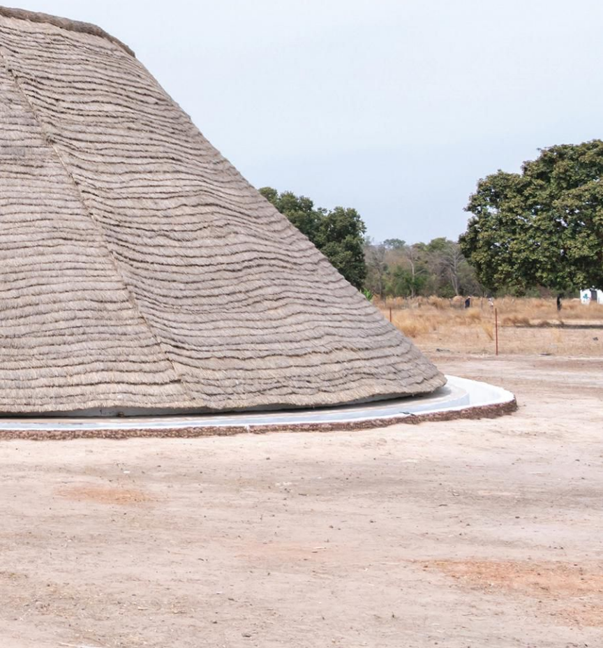
Architect Toshiko Mori borrowed the Fass School's oval shape (left) from an ancient compound in the region. A bamboo and thatched-grass roof dips down over the school structure to provide shade and funnel rainwater (above).
