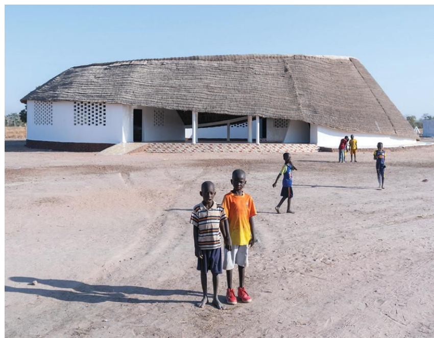
Architect Toshiko Mori borrowed the Fass School's oval shape (left) from an ancient compound in the region. A bamboo and thatched-grass roof dips down over the school structure to provide shade and funnel rainwater (above).
