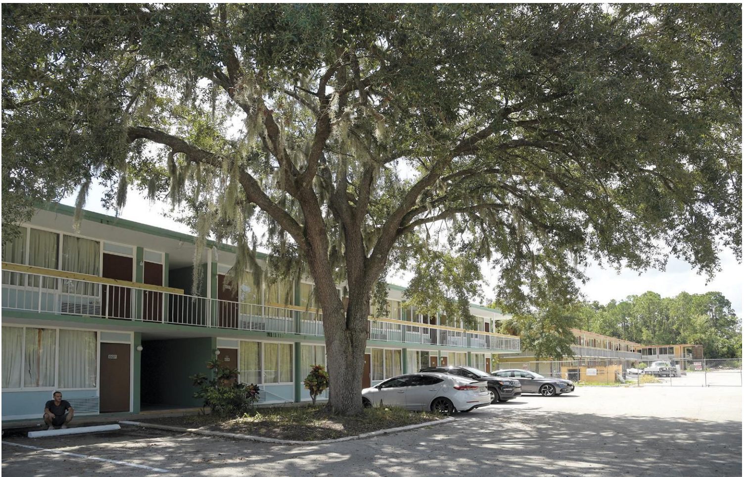
A Travelodge motel on U.S. Highway 192 is being converted into the Backlot Apartments, to provide efficiency housing for working-class renters.
