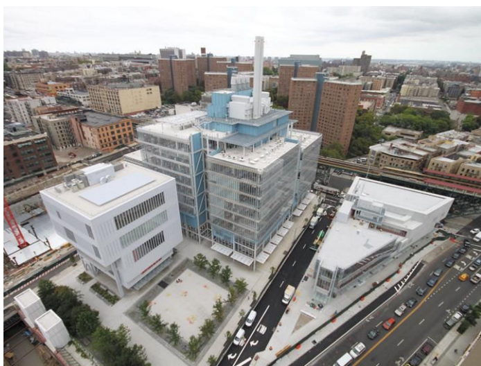
Clustered around a public plaza called the Small Square (left), the Forum (the triangular building) joins the Lenfest Center for the Arts (at left in photo) and the Jerome L. Greene Science Center (in the middle).
