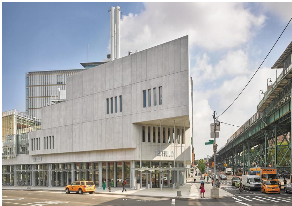
Generous glazing at the street level is meant to give the impression that the Forum is floating. To underscore that idea during the design, Renzo Piano did not include a ground floor in any of his sketches of the building.
