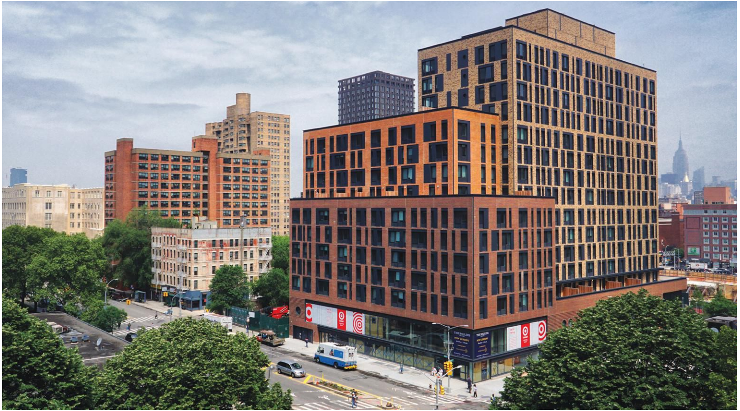
A crop of new high-rise residential towers—including Steiner NYC's 55-story Hub (at left, opposite) by Dattner Architects—is changing the landscape of Downtown Brooklyn and neighboring Fort Greene. The Rollins (above), by Beyer, Blinder, Belle, is a mixed-use, mixed-income residential and commercial building on Manhattan's Lower East Side.
