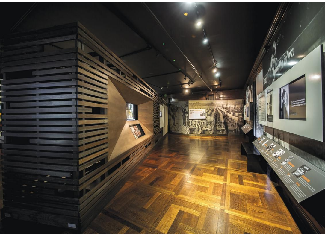
During a renovation, the lighting in the Holocaust Memorial and Tolerance Center of Nassau County was replaced with architectural LED fixtures, including wall washers and monopoints.
