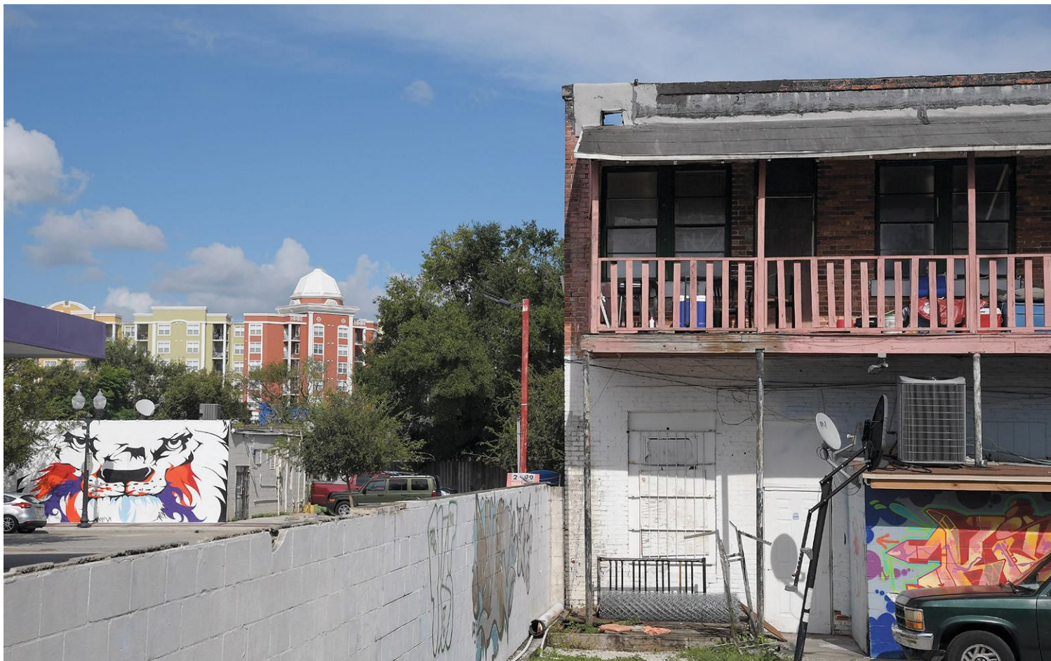
Aging structures continue to provide shelter to families as mid-rise residential buildings sprout up around the city.
