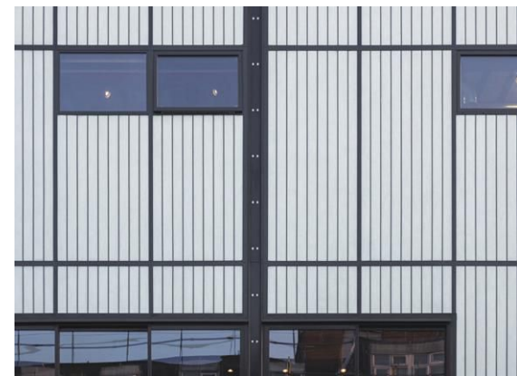
Crouch End Picturehouse | London, UK Unitized Curtain Wall | Adaptive Reuse
