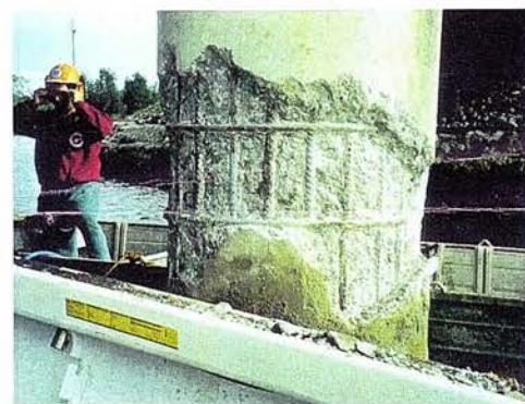
This concrete support has deteriorated due to abrasion and erosion in a tidal zone.
