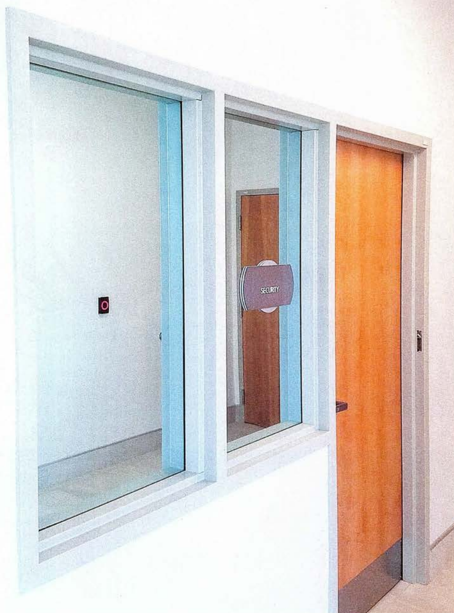
Wood bullet-resistant doors in steel were used in the emergency areas of the 72-bed Major Hospital, a general medical and surgical hospital located in Shelbyville, Indiana.
