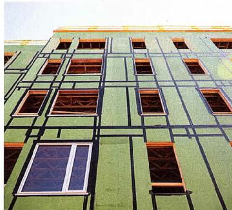
The IBC and IRC codes require a water-resistive barrier behind the exterior cladding plus a means for draining water along that barrier back out to the exterior.
