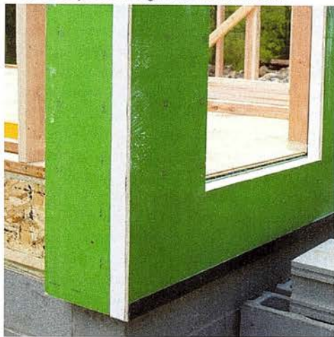
One way to add R-value to wall assemblies is to use single-panel sheathing systems with a built-in layer of continuous foam insulation integral to the back of the panel.
