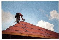
Integrated structural sheathing with built-in underlayment and taped seams for a "sealed roof deck" are used on roof systems as part of sustainability and resilient strategies to help protect against water intrusion, particularly in high-wind-prone areas.
