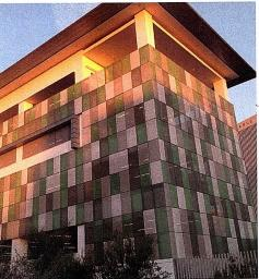
Perforated metal sunscreens can be used on building facades in a variety of ways to help control energy use while still providing light and ventilation as well as biophilic design possibilities.
