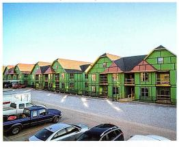
Integrated structural sheathing is available that provides an integrated water barrier and air barrier with tape-sealed seams, which streamlines installation and can help improve long term performance.
