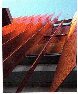
to keeping the building cooler in the sunlight, perforated metal can also allow controlled light and views either directly through perforations in the sunscreen or between vertical louvers or baffles. There are also any number of other creative design options for daylight and views with this material based on the needs of the building and the overall design intent.
