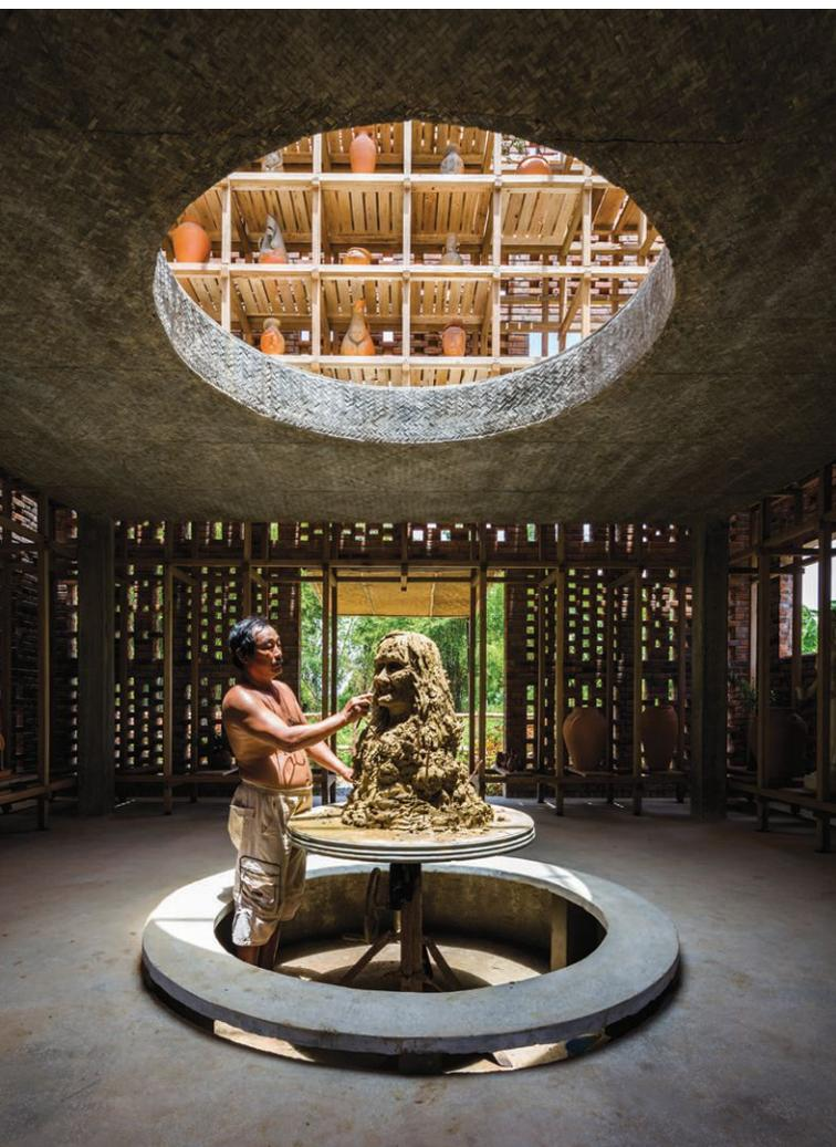
**BEHIND THE VEIL** Inside the two-story ceramist's studio, a stout 16-inch-thick slab is supported on four concrete columns (above). Between this slab and the exterior brick screen, a timber frame extends to a second level and to the building's glass roof (right), housing stairs and shelves for display.
