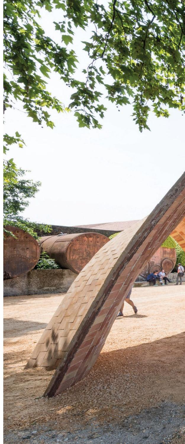
less," the architects worked with engineers from Cambridge, Massachusetts-based Ochsendorf DeJong and Block (ODB) early in the process to optimize the structure. Because the materials for making brick are readily available in Africa, the team decided to explore using an unreinforced masonry system.
