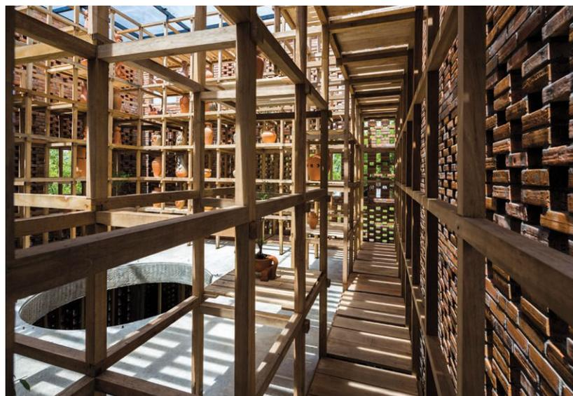
of openwork panels. Each wall is divided into 36 squares made up of several patterns of brick screens with various levels of transparency—created by leaving voids in the brickwork—fitted like patchwork pieces to make the larger square.
