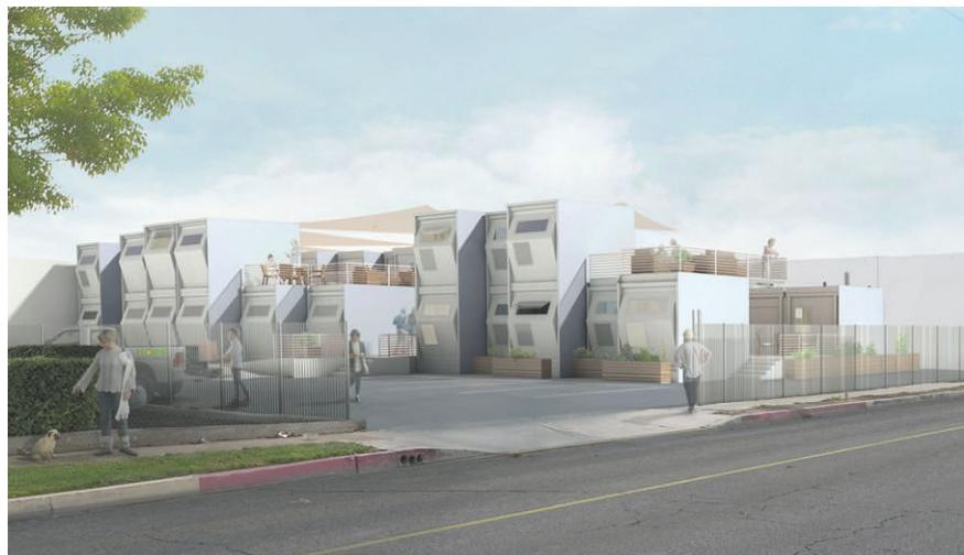
Individual units (left) form stacks that would face inward to an open courtyard (above). The second level is accessible via prefabricated stairs. Each unit is wired for electricity that will tap into the existing grid. Kitchens and bathrooms would be separate, communal structures.
