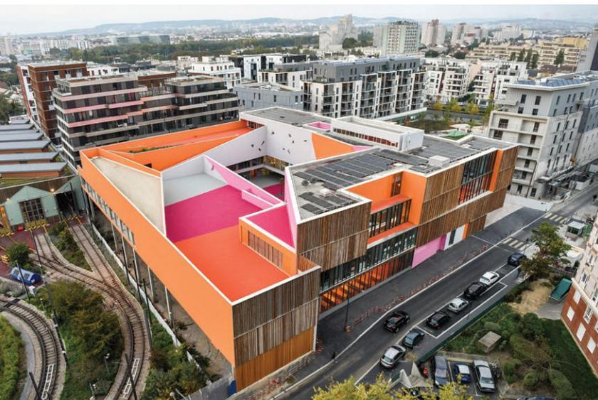
**SMART MOVES** To minimize disruption from an adjacent tramway depot, teaching space is concentrated in the northern part of the building, and a two-tiered elementary school yard occupies the upper floors to the south. Walls enclosing the yard are angled to maximize daylight penetration into the central courtyard.
