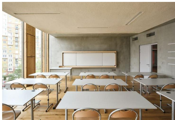
walls create unfolding sequences of compression and release along the routes. The plan varies from floor to floor, so the poured-in-place concrete walls do not vertically align, and loads are transferred through the slabs. Such irregularity is typically expensive, but the building was relatively economical at \$200 per square foot.
