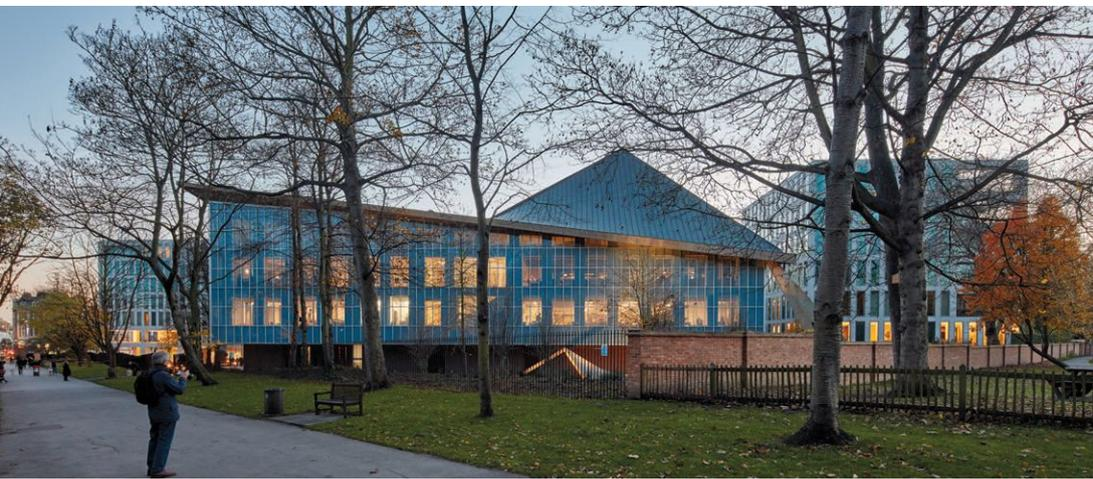
Replacement glazing admits daylight and views to spaces such as the second-floor restaurant (above), but maintains the outward appearance of the original opaque, blue-glass facades during the daytime. At night, the fritted glass allows electric light to seep from the building (left).
