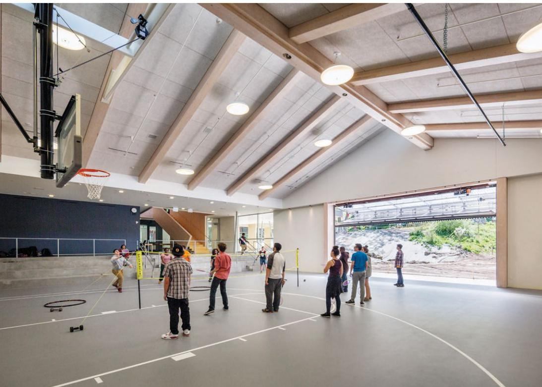
**FAST TRACK** The building's structural components, including glulam beams that frame the roof over the gym (above), and the CLT panels used in the ceiling of a science classroom (top) and a central stair (opposite), were shipped to the site already fabricated and cut to size, accelerating construction.
