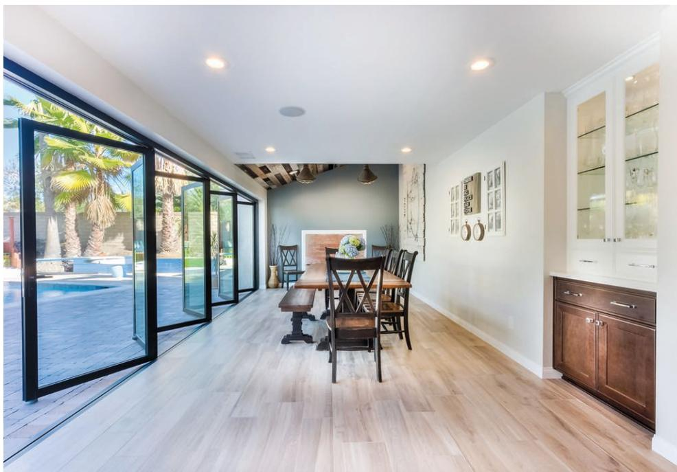
An aluminum thermally controlled folding system in bronze anodized finish with a flush guide sill offer a seamless transition from inside to outside, creating an open-air dining area.
