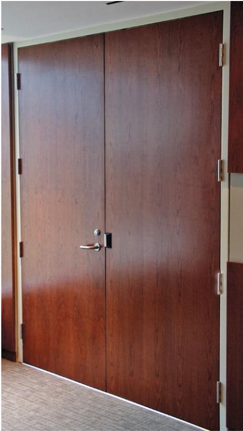
Acoustic wood doors in a steel frame all coordinated and supplied by a single manufacturer can be carefully controlled and tested to achieve high performance, such as this door that is verified at STC 51.
