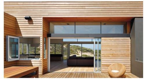
Aluminum pocketing multi-slide system spanning a 15-foot-wide opening.
